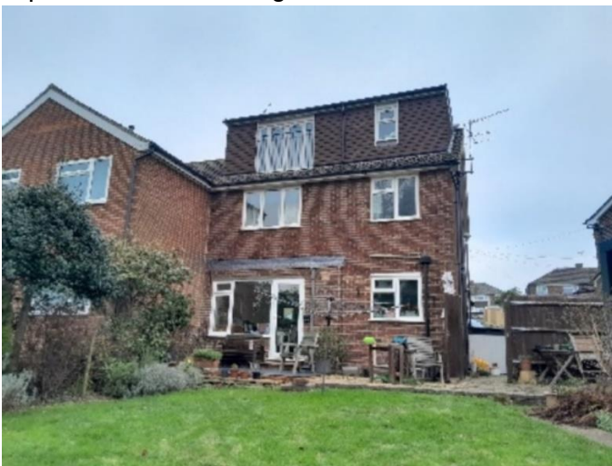
Fig 1: View from the rear of the property (17/02/25)
