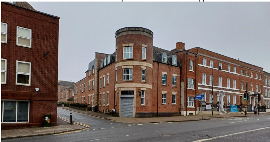
View of the application site building from London Street
