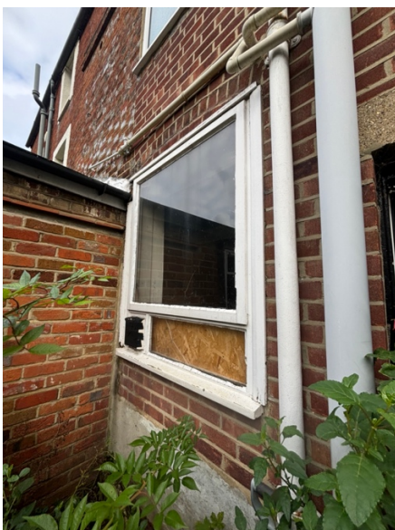
Photo showing the ground floor rear window, to be replaced.
