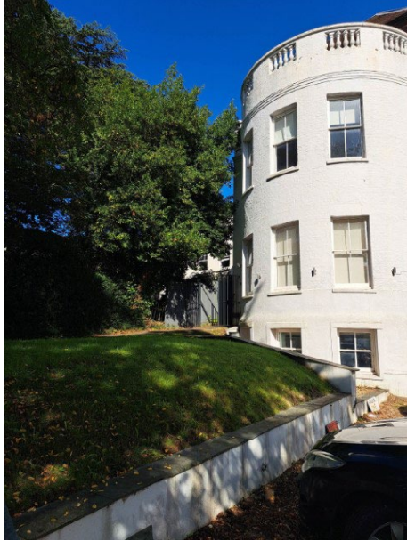
Photo 9 – View of the security gate and fence from a south-east elevation
