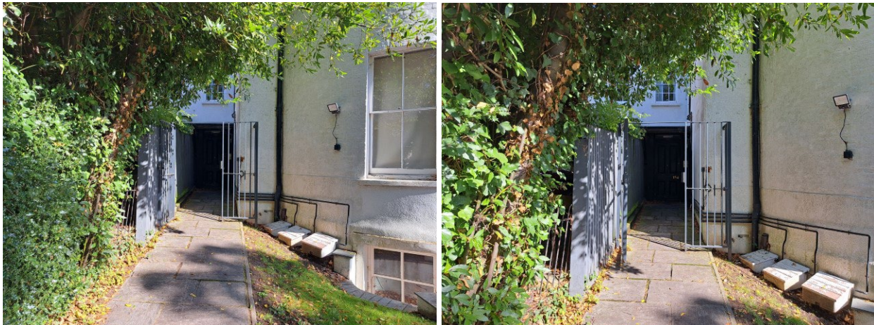
Photo 2-6 – View of the security gate and fence from a south and north elevation
