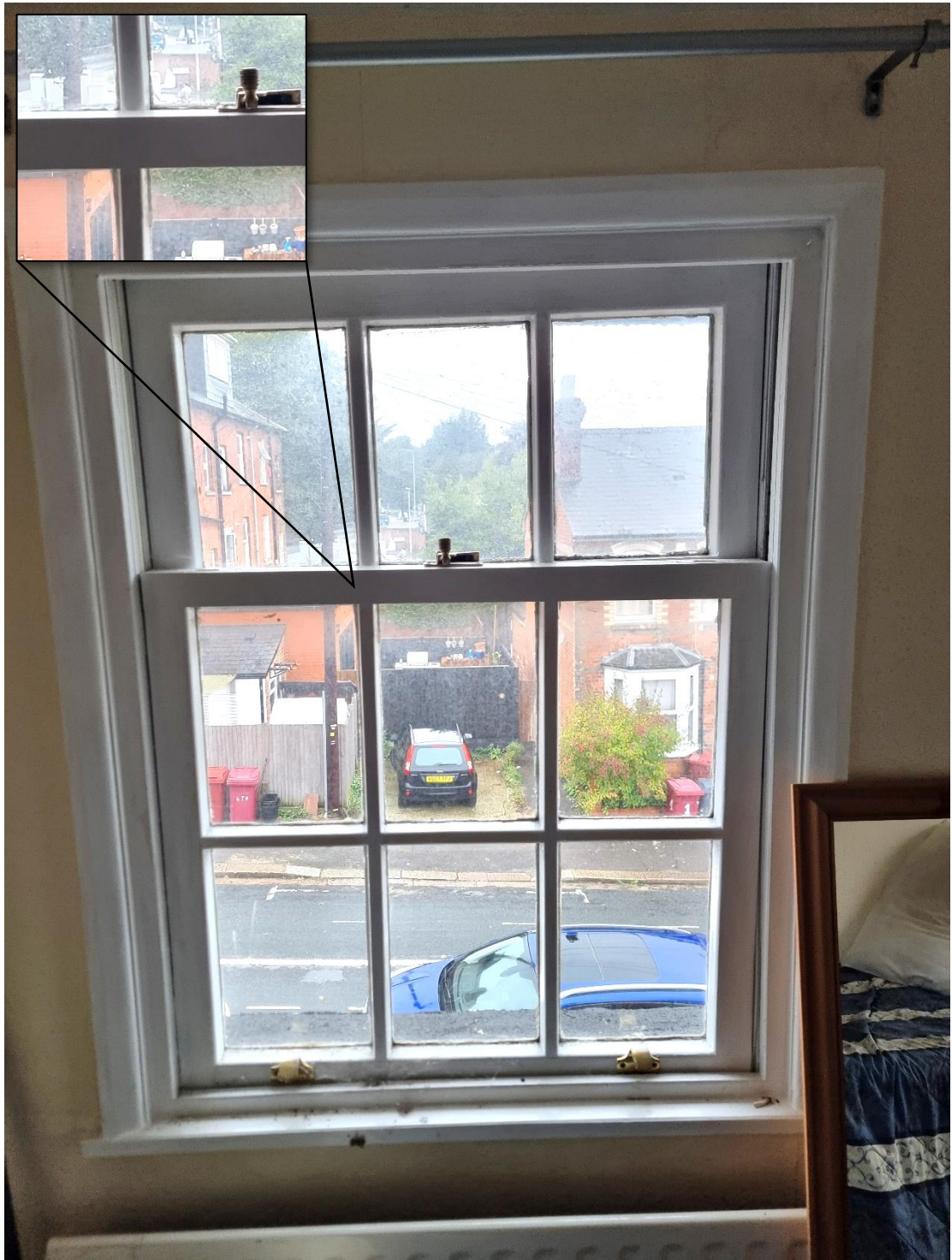
Fig.23: Example of modern replacement window (first floor northwest bedroom), identified by thick, square profile glazing bars.
