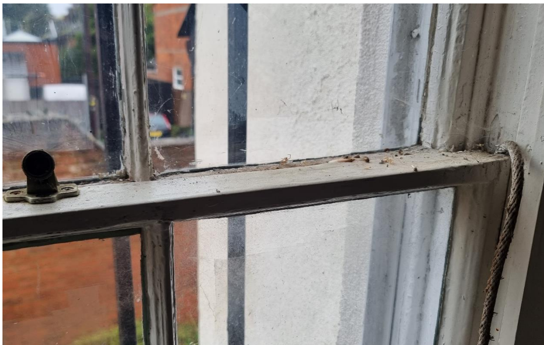
Fig.26: Detail to historic sash window.
