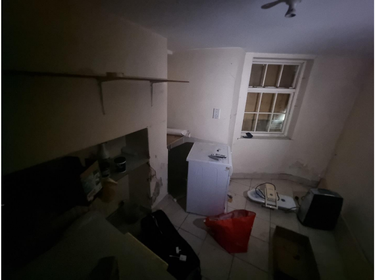
LGF11 – Modern fabric and replacement window. Former window to right blocked up and split by modern partition
