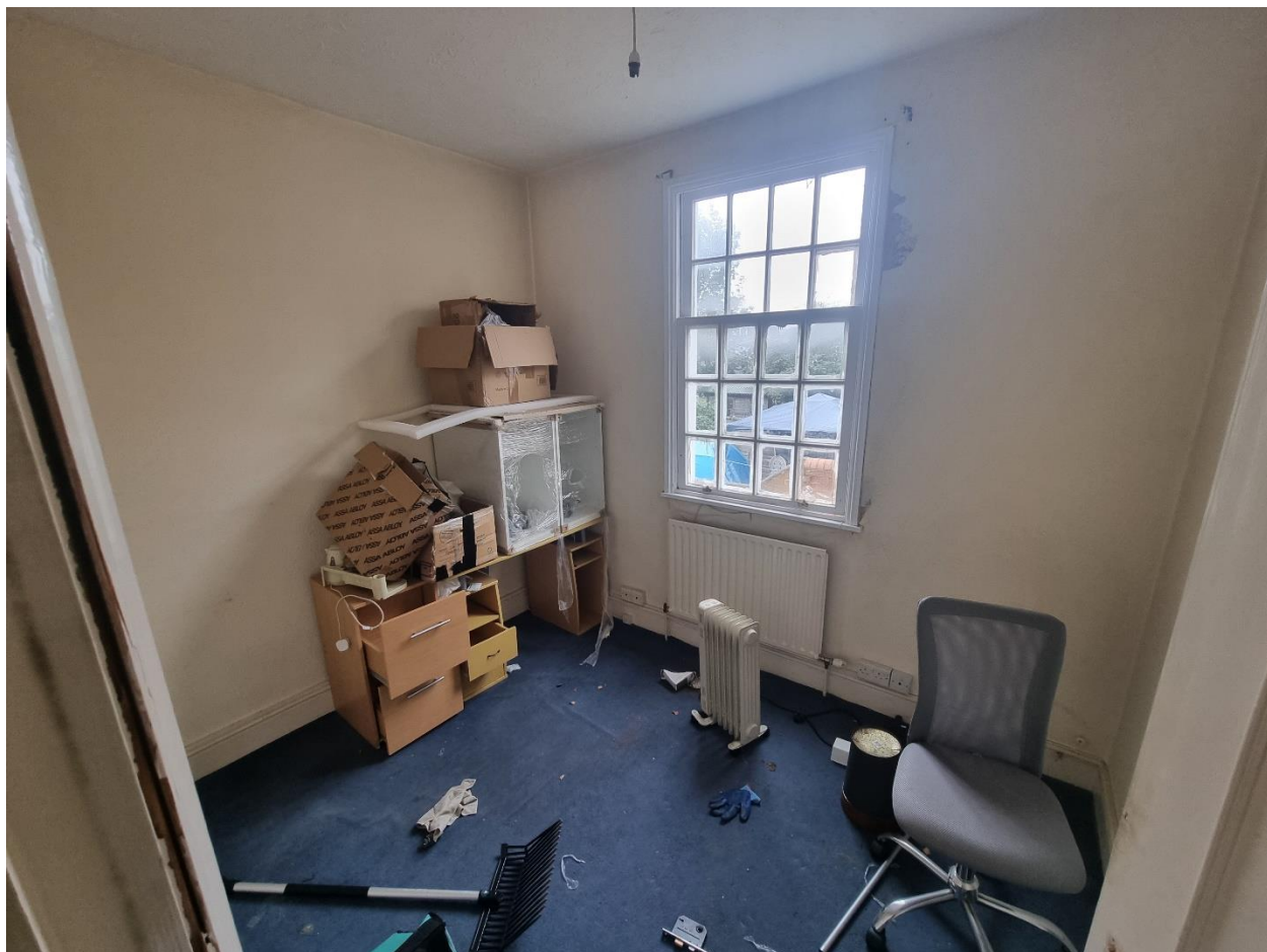
GF9(2) – Former window to left infilled internally (sealed and painted over externally)
