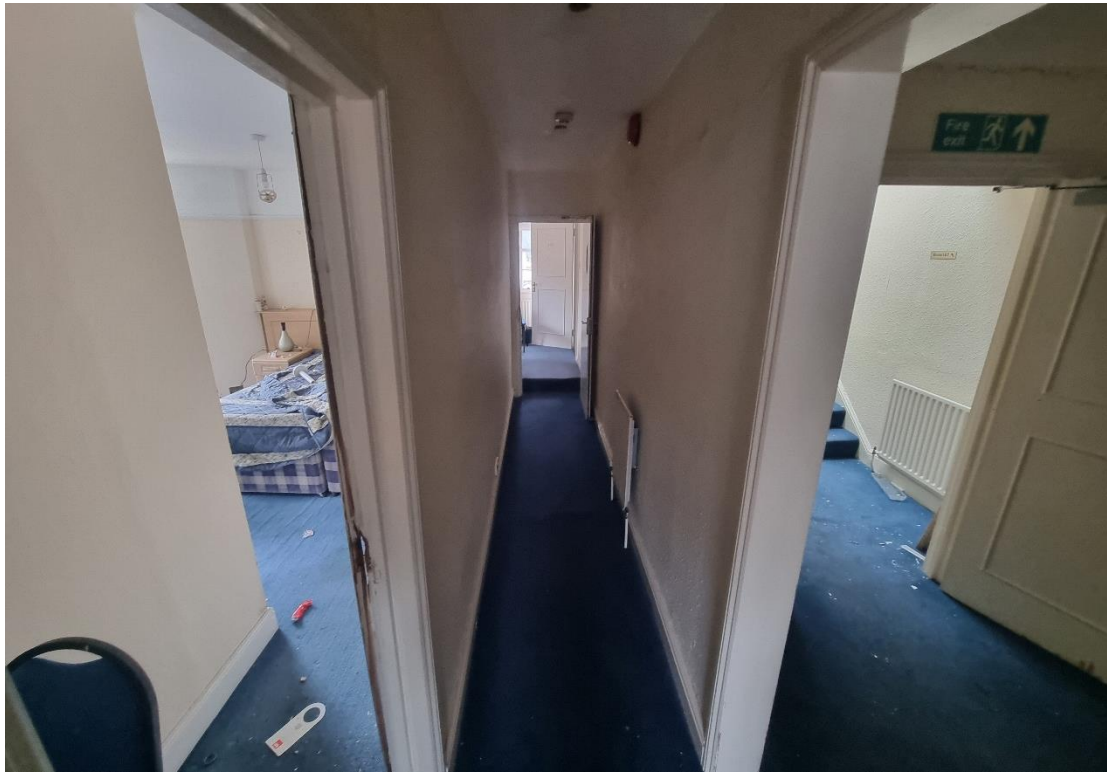
Fig.13: Example of narrow post-construction corridor (seen here to first floor, south side) with modern partition in front room to left and stairwell to right.
