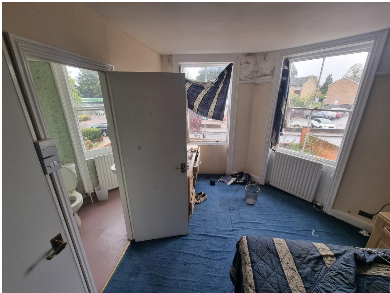
FF6(1) - Early 20 th century replacement windows with modern single glazing (non-original but mentioned in 1976 listing), surround with possible historic context, modern partition
