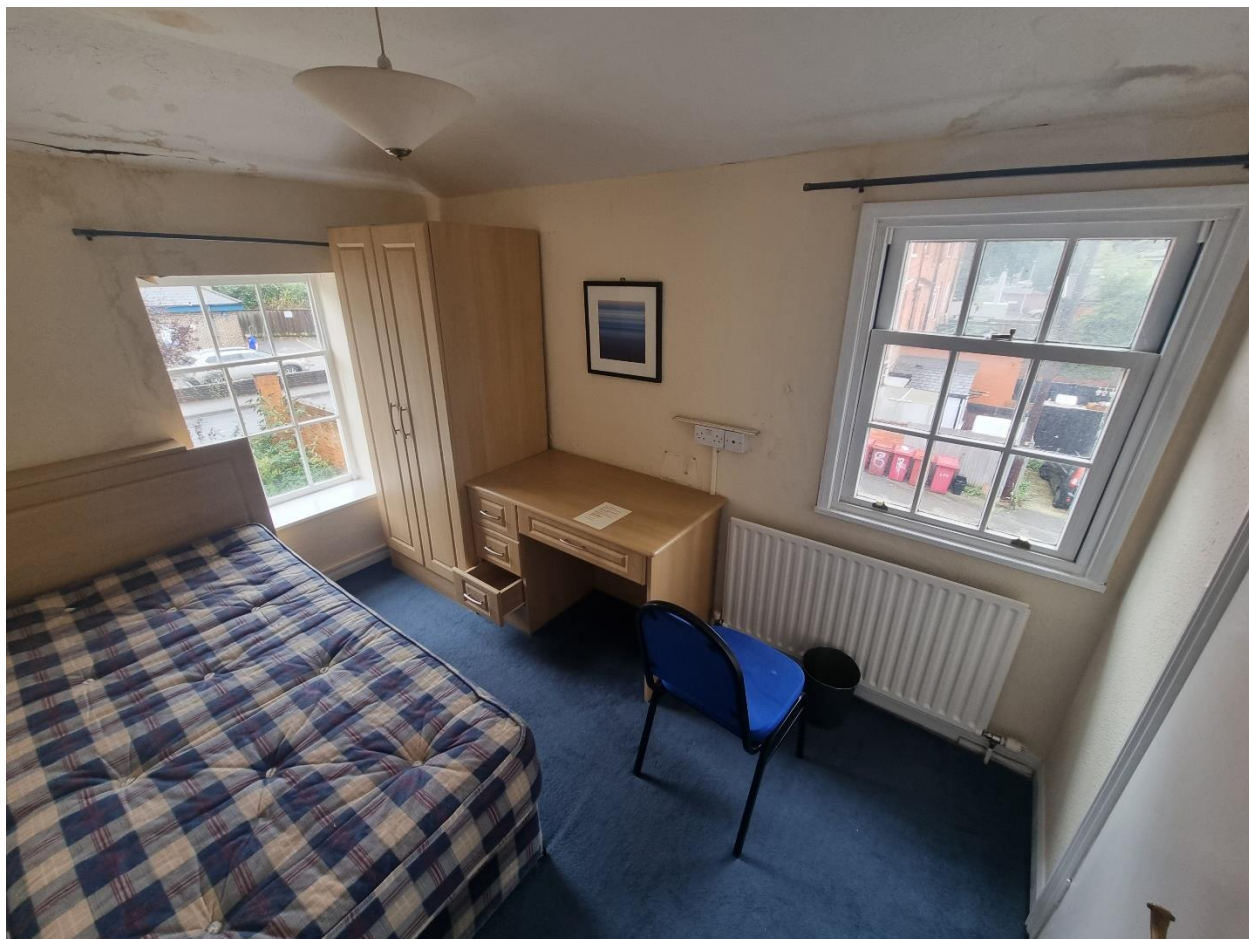
FF8 – Modern fabric and windows
