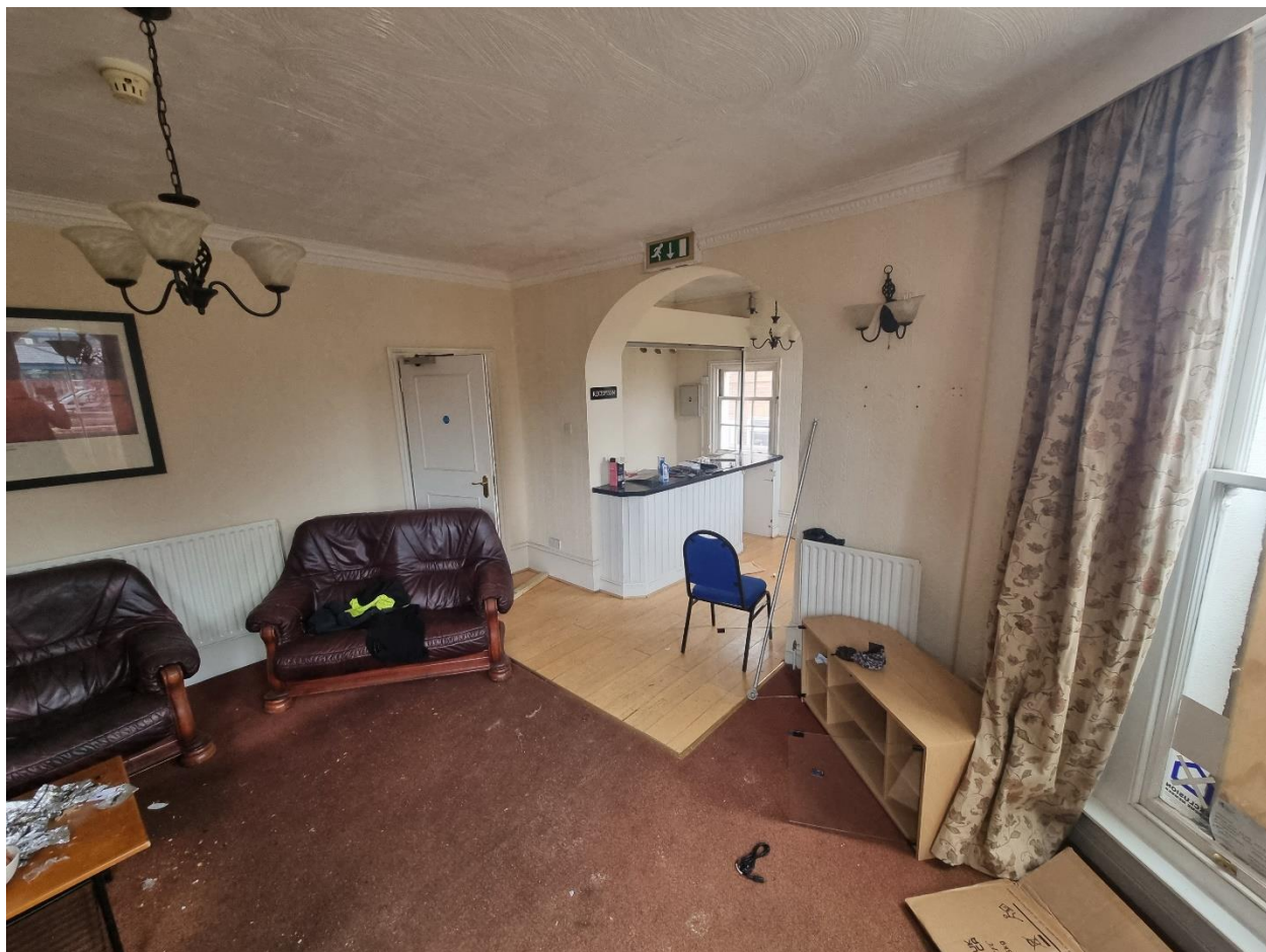
GF2(1) - Mixed context historic and replacement skirting and cornice, post-construction alteration to arch
