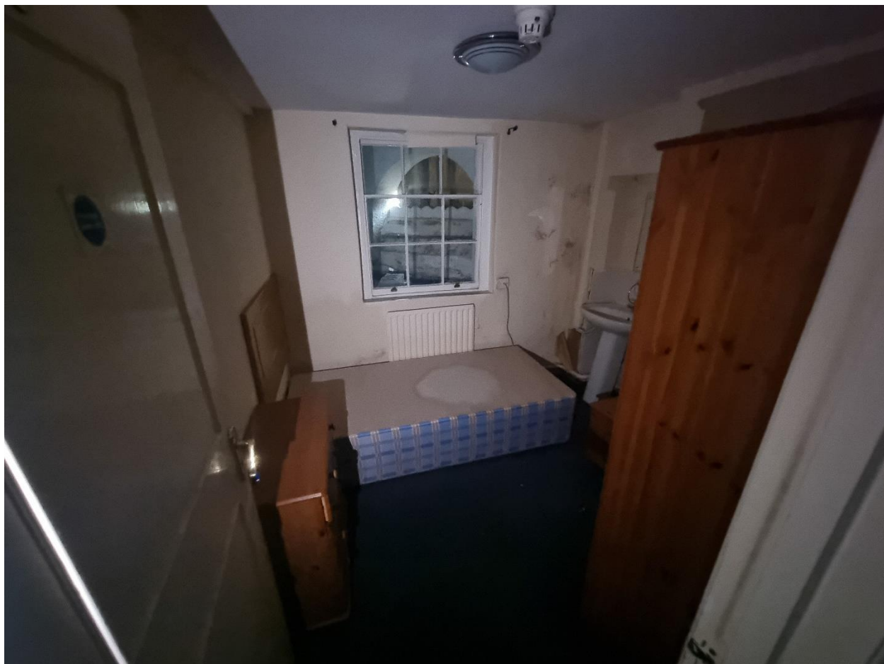
LGF8 – Historic window with replacement modern glazing
