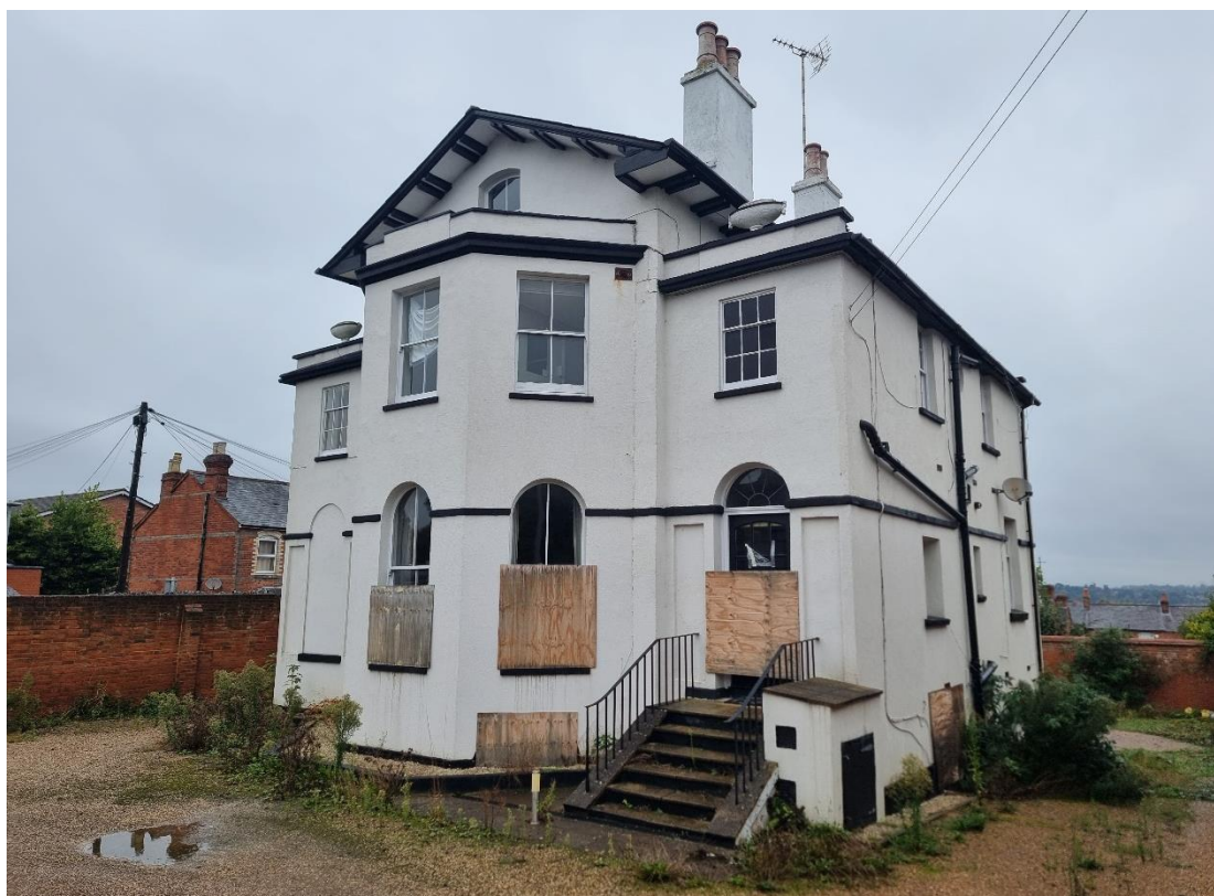
Fig.27: 2 Tilehurst Road after the closure of 'Belle Vue House Hotel' (c.2020).
