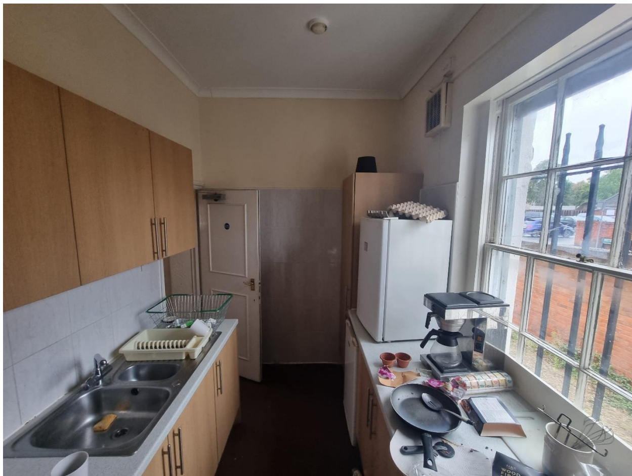
GF3 – Modern fabric, historic window with modern single glazing
