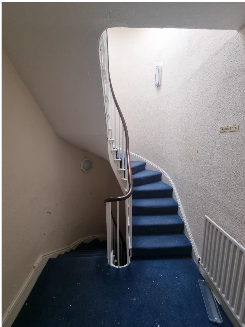
FF1 – Historic stairs and skirting, modern textured finish
