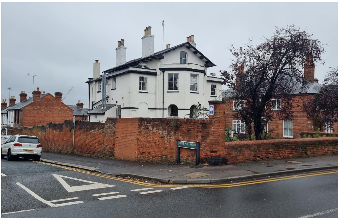
Fig.3: The property seen from the corner of Tilehurst Road and Belle Vue Road.
