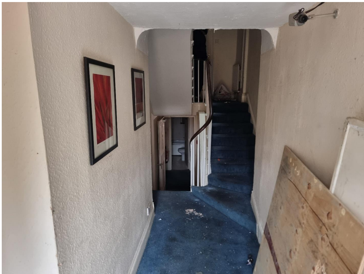
LGF1 – Historic stairs, modern wall finishes
