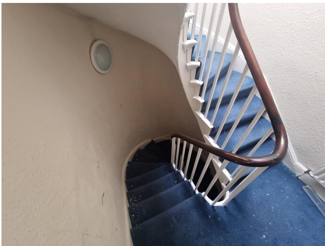
Fig.16: Stairs with historic context including balusters, bannisters, and skirting. Walls refinished with modern textured plaster.
