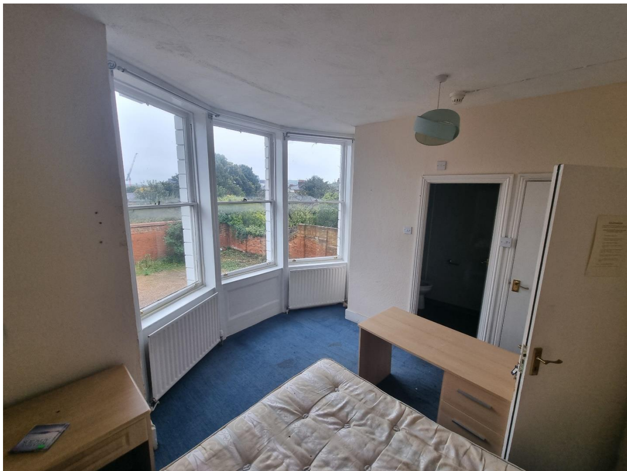
GF6(1) – Modern fabric and ensuite partition, early-mid 20 th century replacement windows
