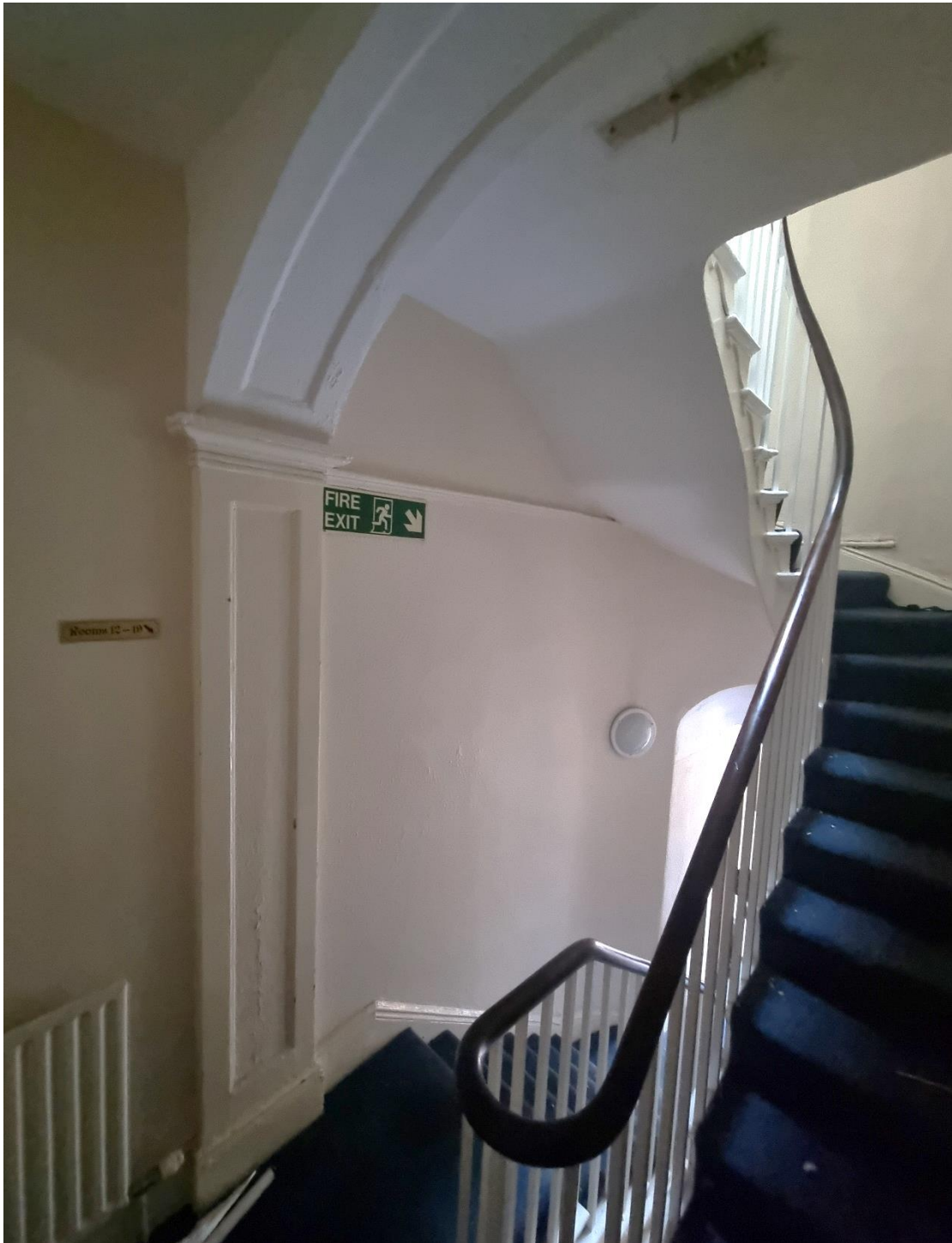
Fig.17: Ground floor stairs landing with arch of historic context.
