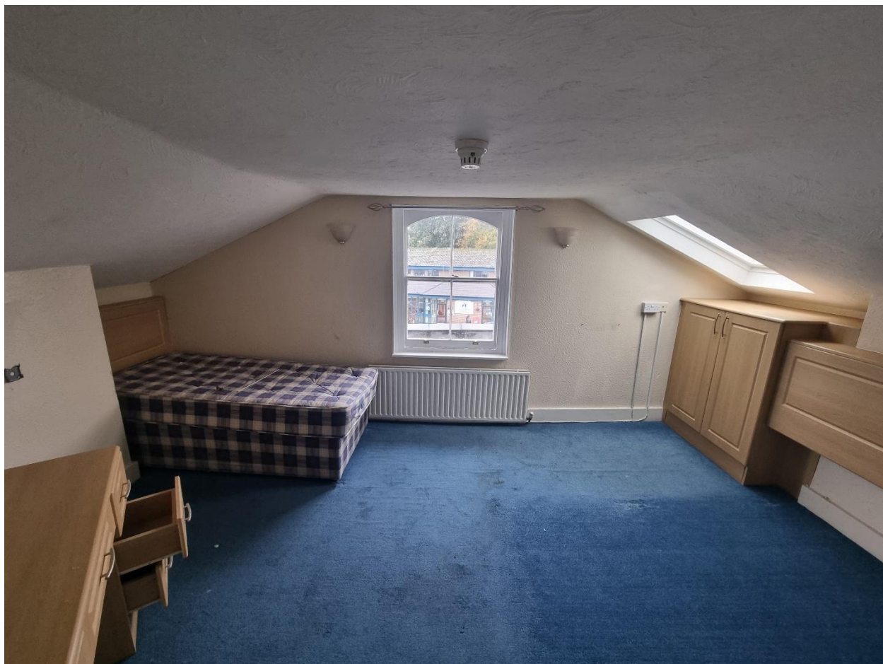
SF3(1) – Modern fabric, early 20 th century replacement window with modern glass
