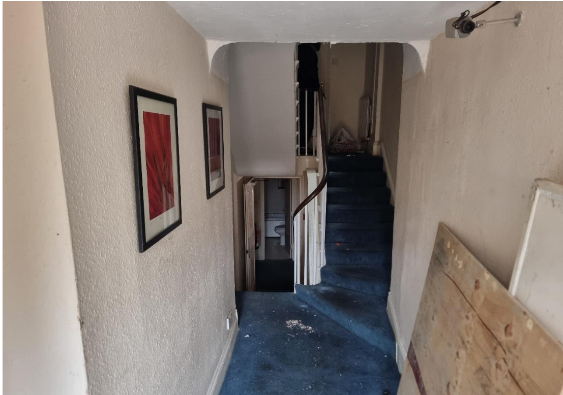
Fig.20: Stairs and landings to lower ground and ground floors, seen from the side entrance.
