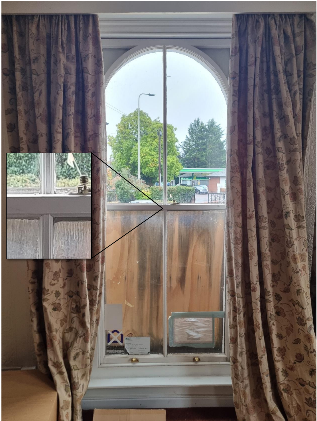
Fig.24: Example of early/mid-20 th century replacement windows (typically found fitted to canted bays, as here to ground floor lounge) with larger individual panes and clean, machine-cut glazing bars.
