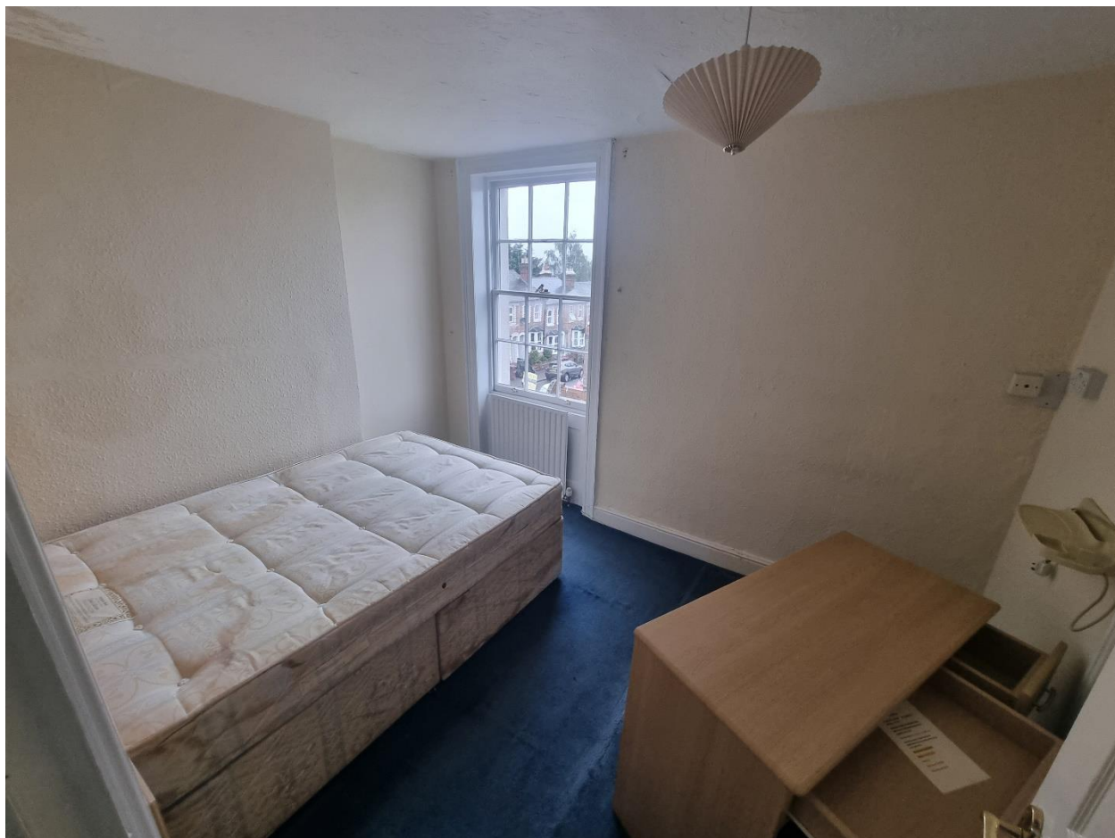
FF13 – Historic window to left with modern single glazing, former French door to centre infilled internally (sealed and painted externally), modern fabric
