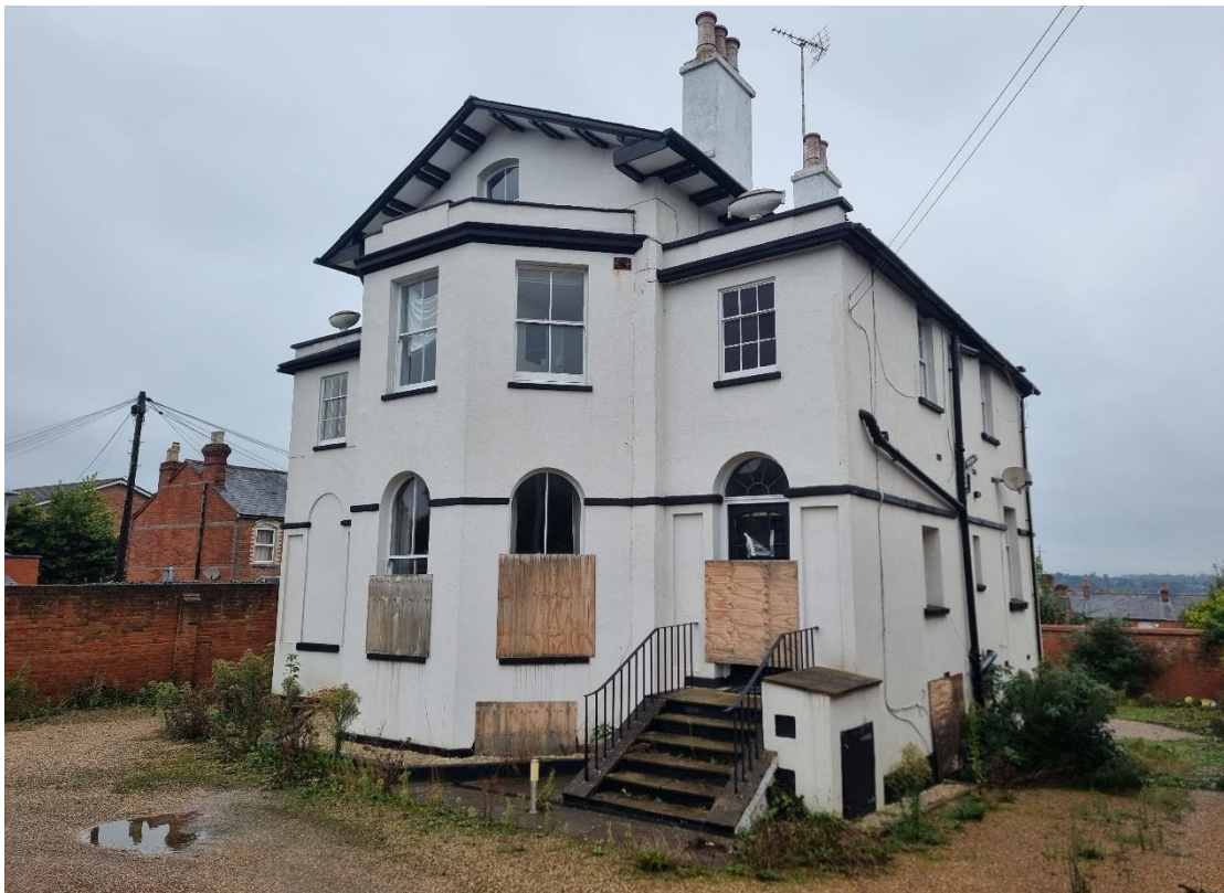
Fig.5: The front door of the property, secured along with the accessible windows to prevent persistent trespass issues. The first floor window over the door has been infilled internally and the panes painted black. The entirety of the site is laid with gravel and is currently overgrown due to prolonged vacancy.
