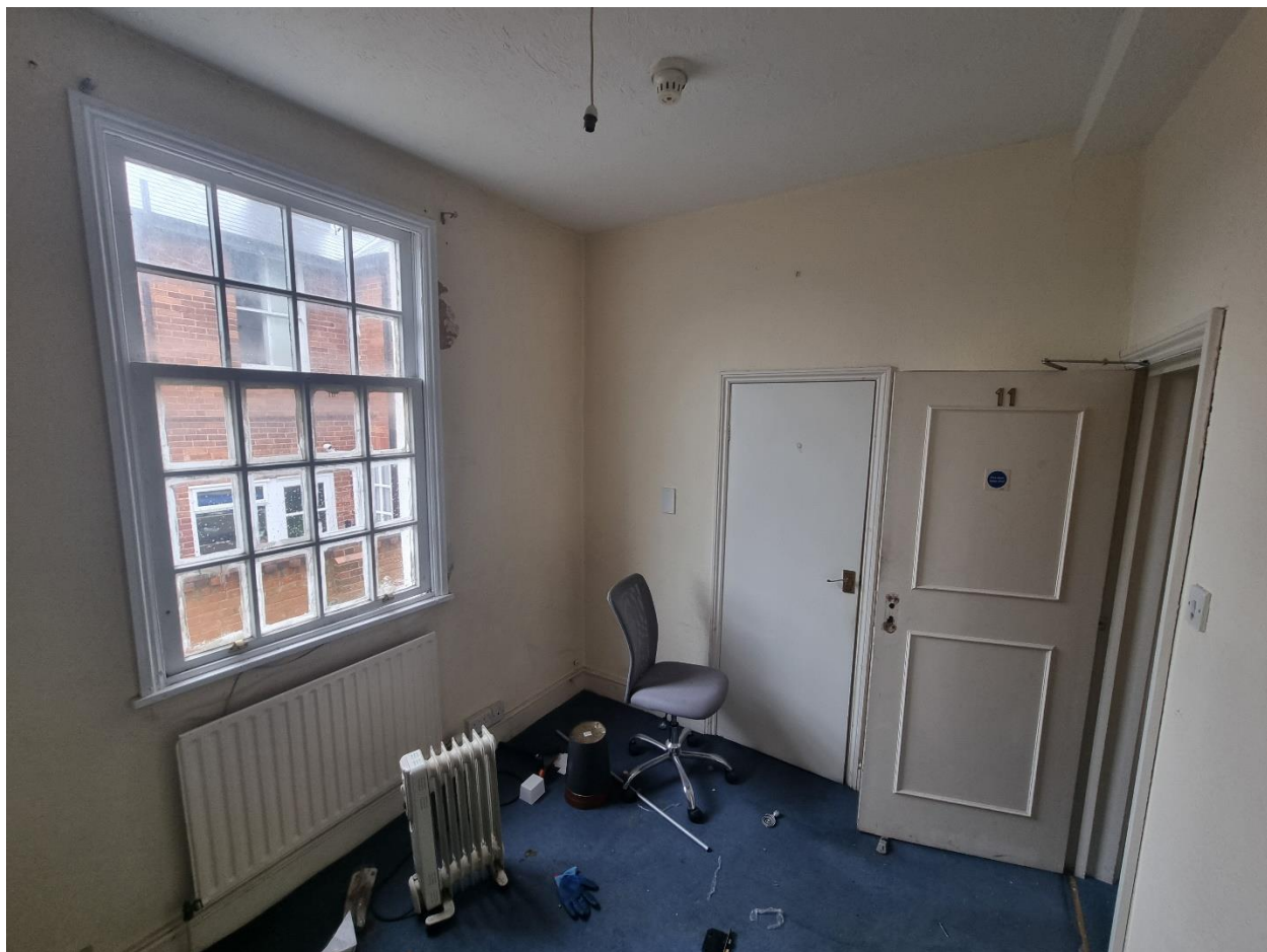
GF9(1) – Modern fabric and window
