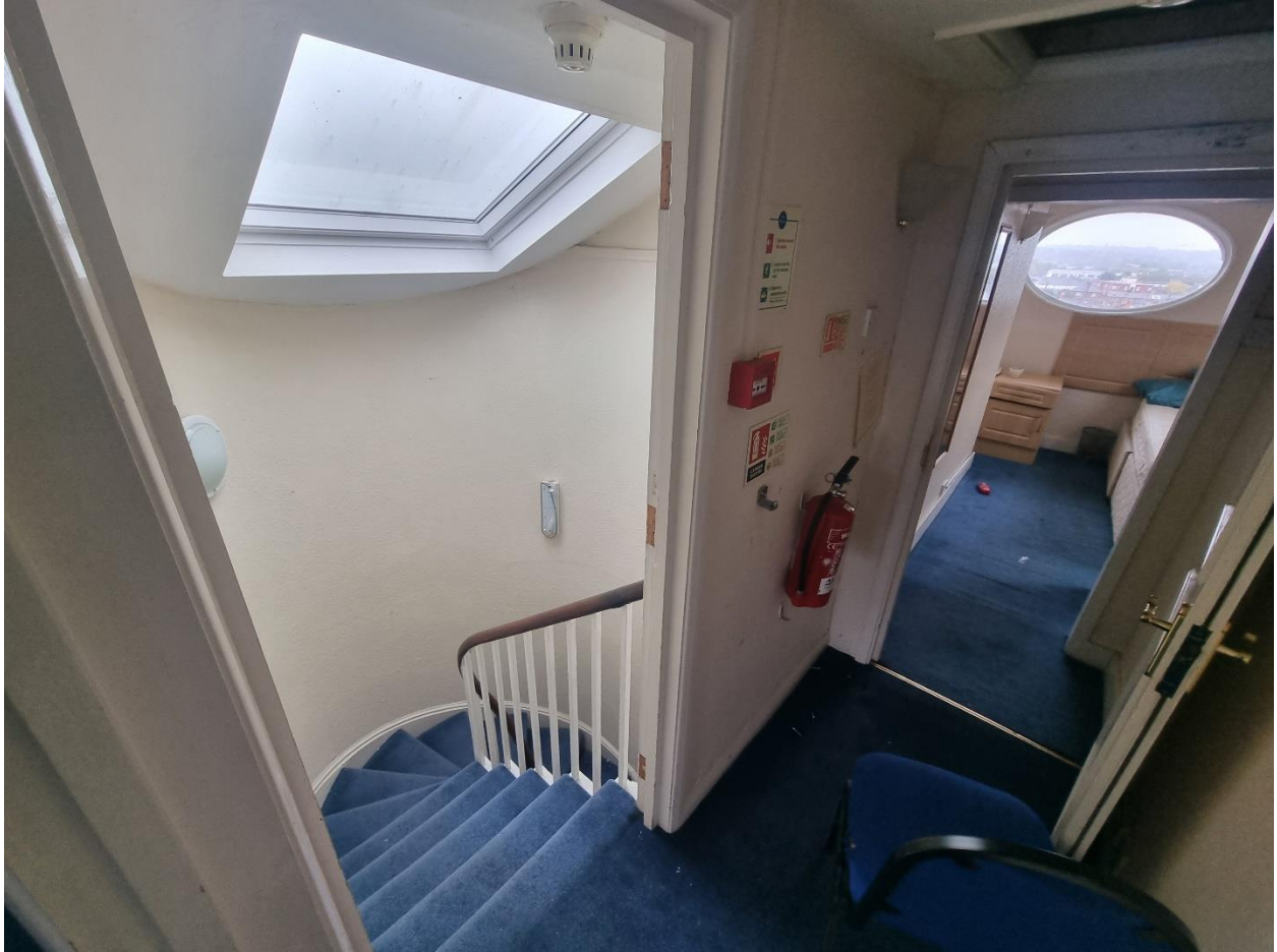
SF2 – Modern fabric including wall, skylight, ceiling hatch, and doors
