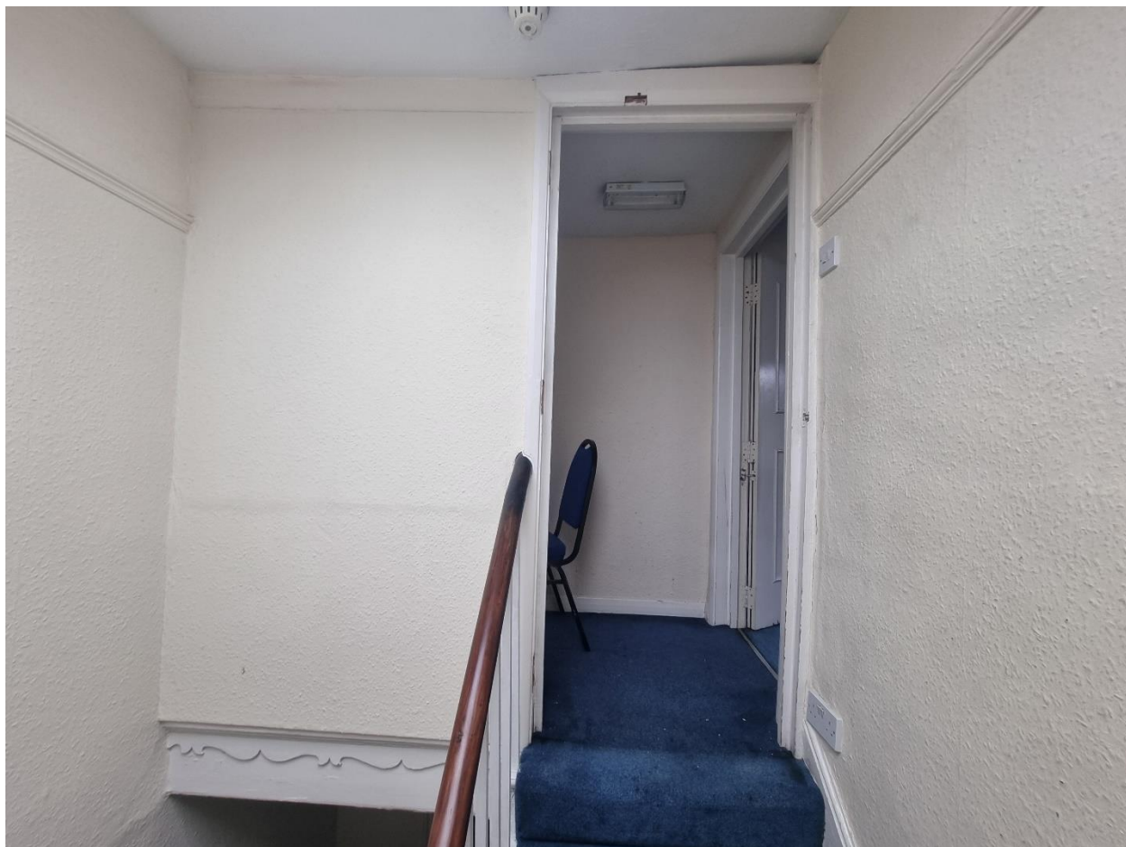
SF1 – Historic stairs and detailing, modern textured wall finish and ceiling
