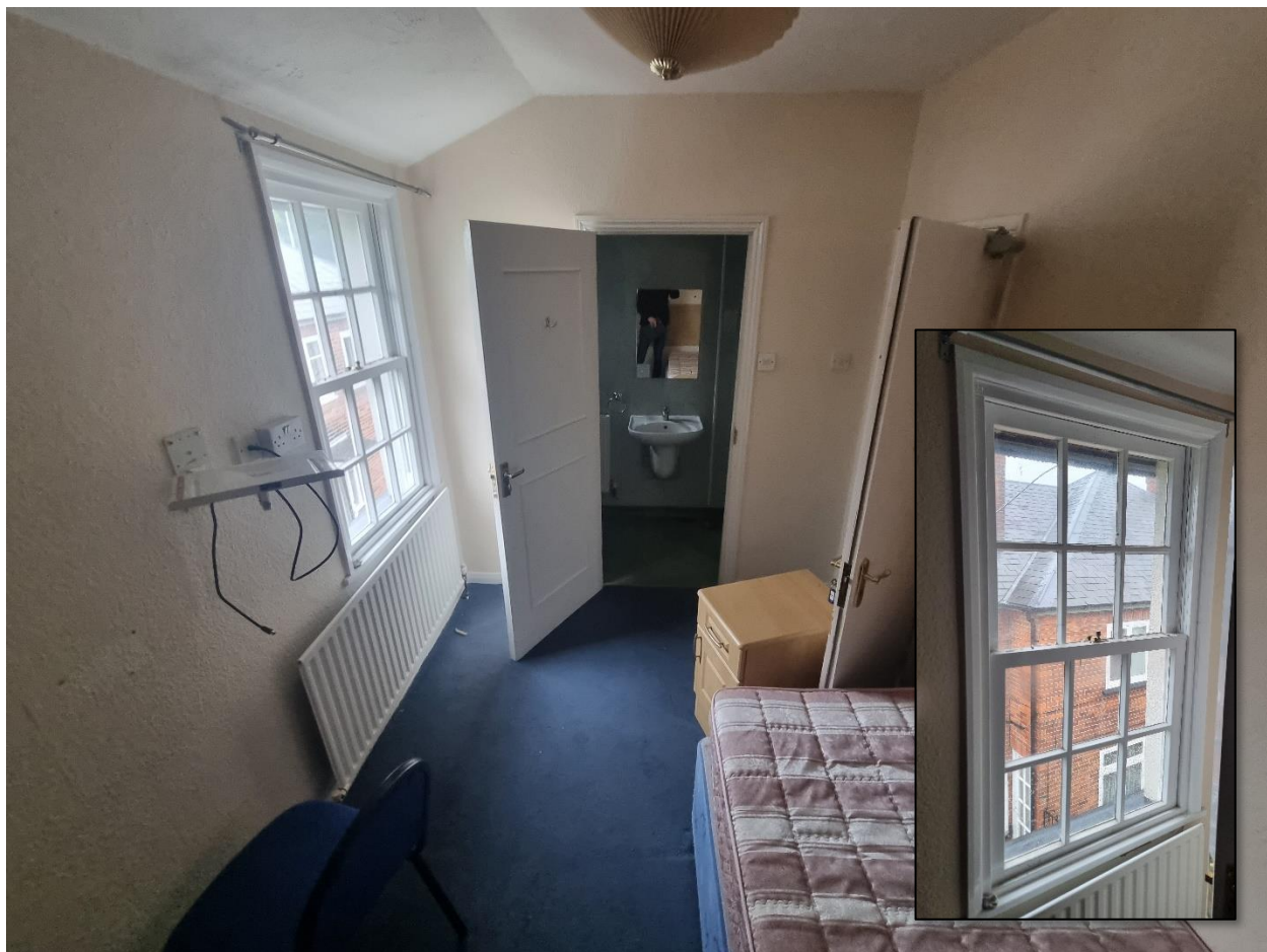
FF15 – Modern fabric and window (inset), additional infilled window behind camera
