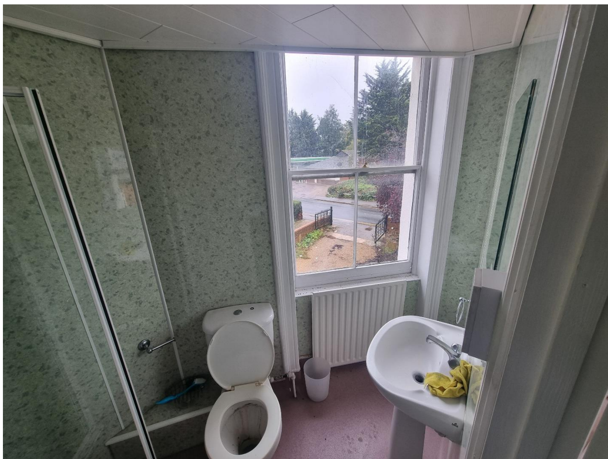
FF7 - Early 20 th century replacement window with modern single glazing (non-original but mentioned in 1976 listing), surround with possible historic context, modern partition and lowered ceiling
