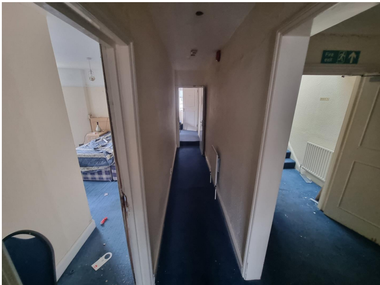
FF5 – Modern fabric and partitions
