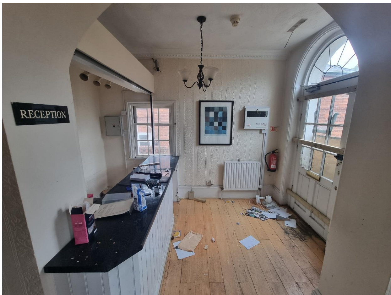
GF1 – Mixed context historic and replacement skirting and cornice, modern door with historic fanlight, modern sash window
