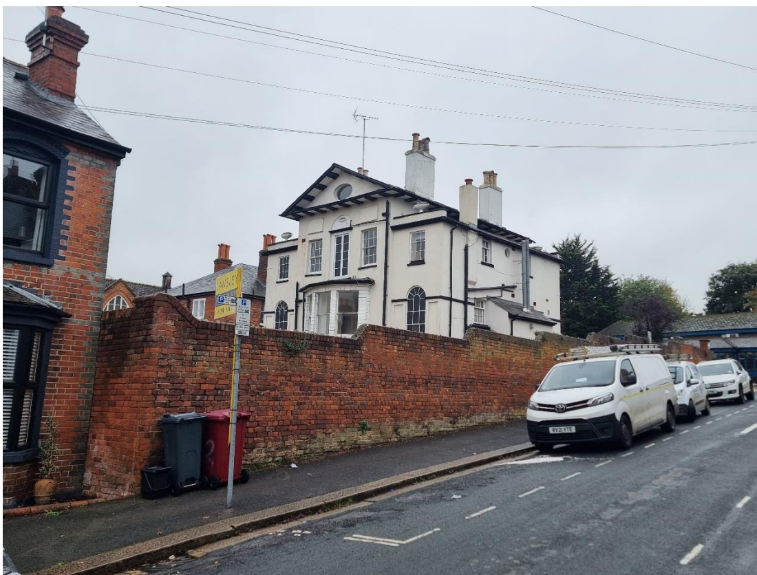
Fig.4: Rear (north) elevation of the property seen over the wall on Belle Vue Road.
