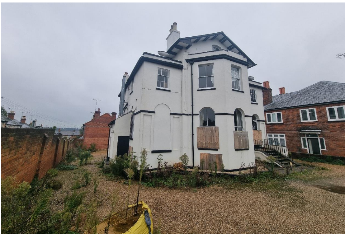
Fig.6: Looking along the west side of the property towards the rear. The arch to the opposing side to the front door is blind and may be a post-construction infill.
