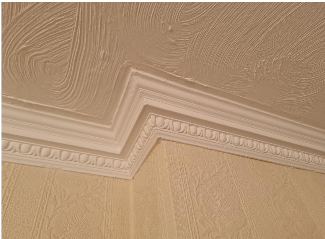
Fig.19: Cornice detail (lounge and reception) plus modern texture and papering to ceiling and walls.
