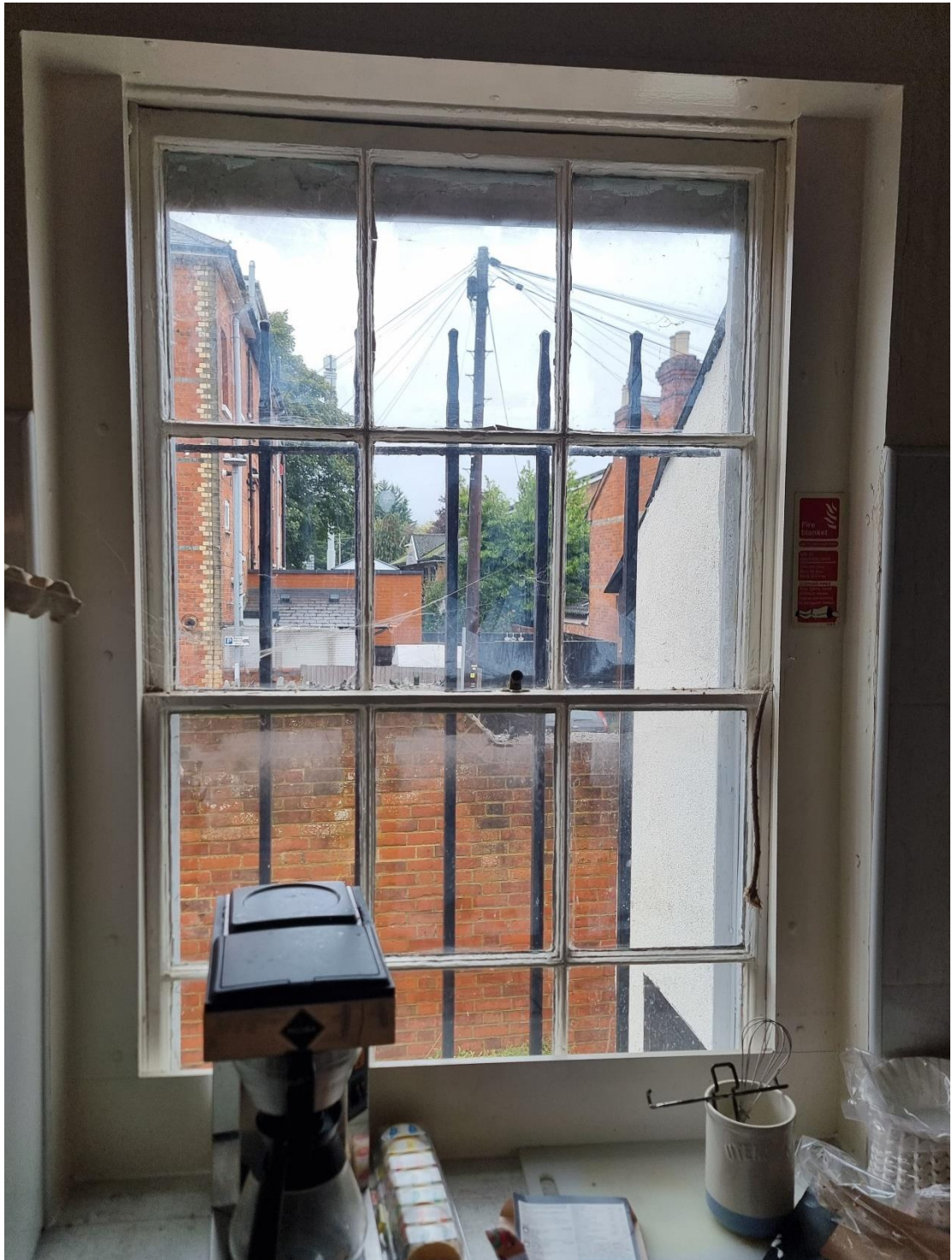
Fig.25: Example of a retained historic sash window (ground floor kitchen), though all identified examples include modern replacement single glazing and further interventions. Characterised by thin profile glazing bars with pronounced wear and lack of horn braces.
