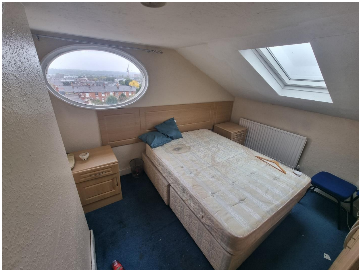
SF4(1) – Modern fabric, oval window opening of historic context with swivel opening replaced by modern fixed pane glass
