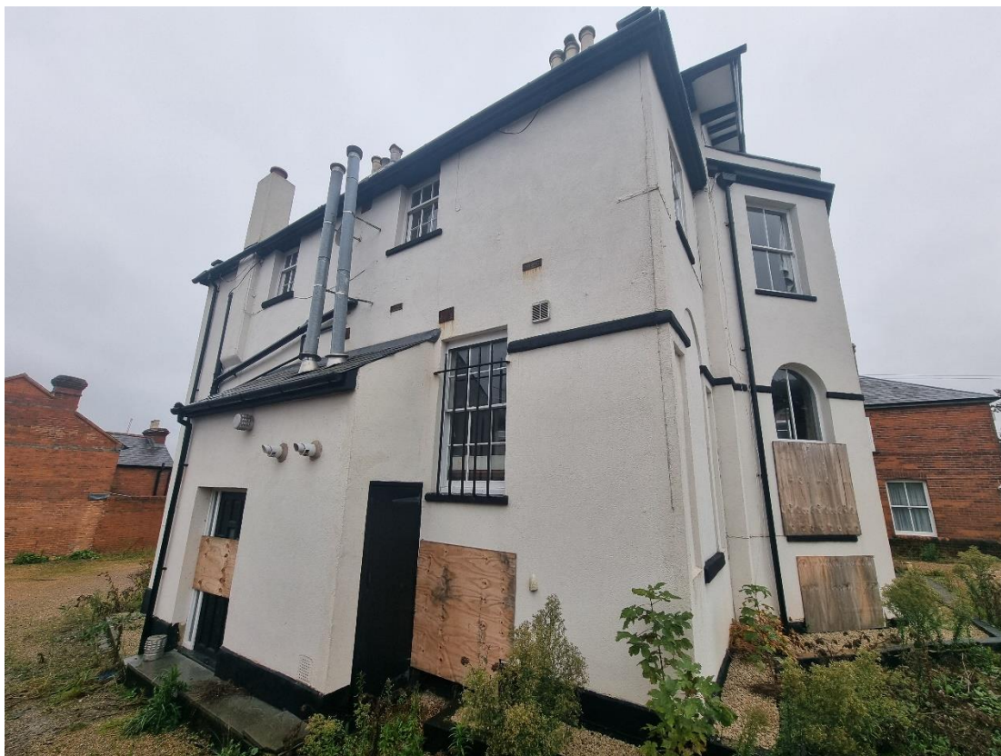
Fig.7: Side access addition to the west side of the property.
