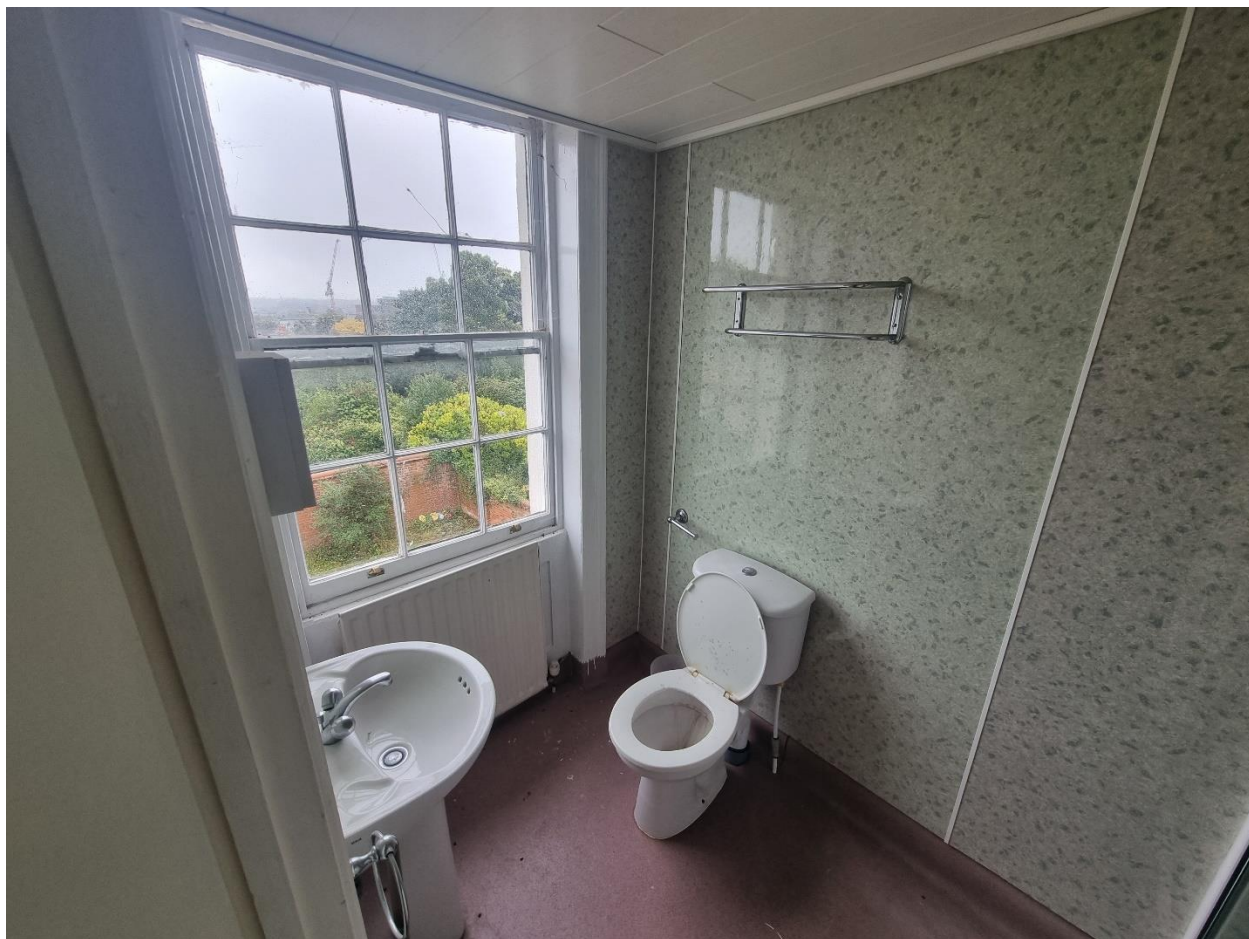
FF14 – Historic window with modern single glazing, modern fabric
