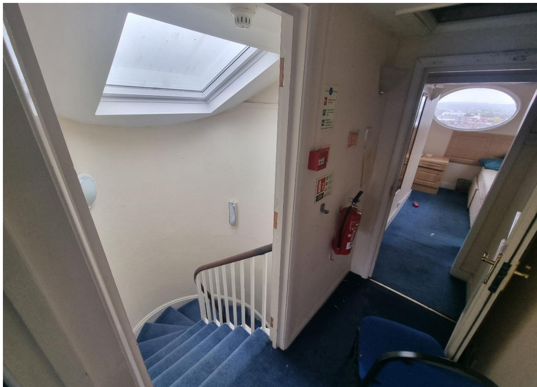
Fig.12: Attic landing, back room with altered historic window (fixed pane set in historic swivel opening frame), and stairwell with modern rooflight.
