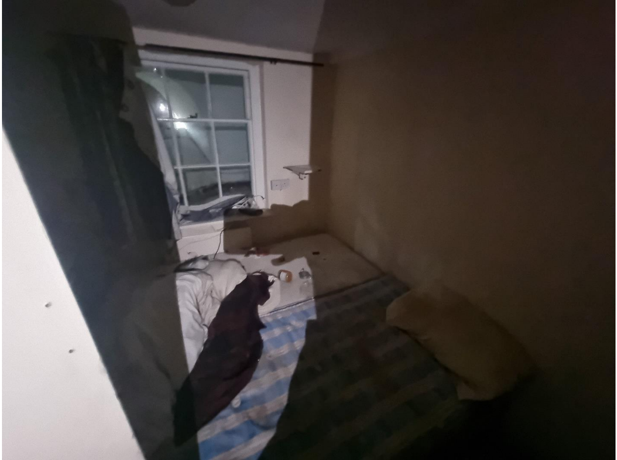
LGF7 – Historic window with replacement modern glazing
