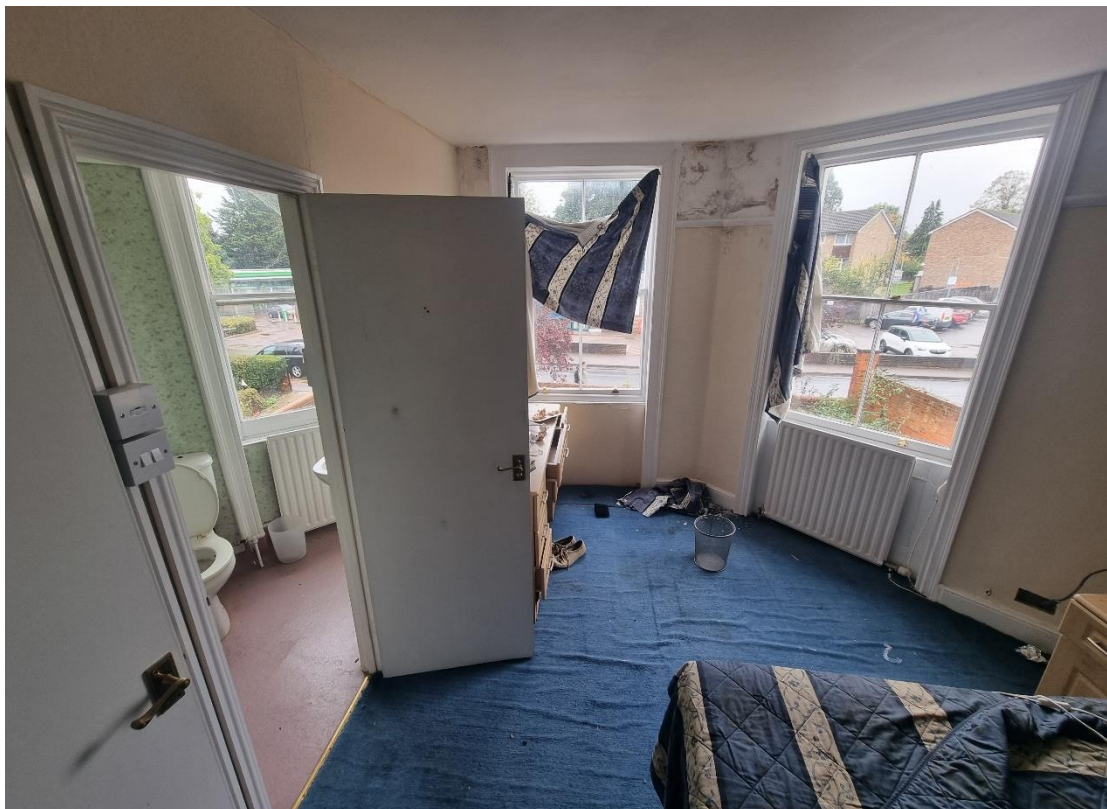
Fig.14: Studwork partition to large first floor front bedroom to form ensuite. Early/mid-20 th century replacement windows, surrounds possibly of earlier historic context.
