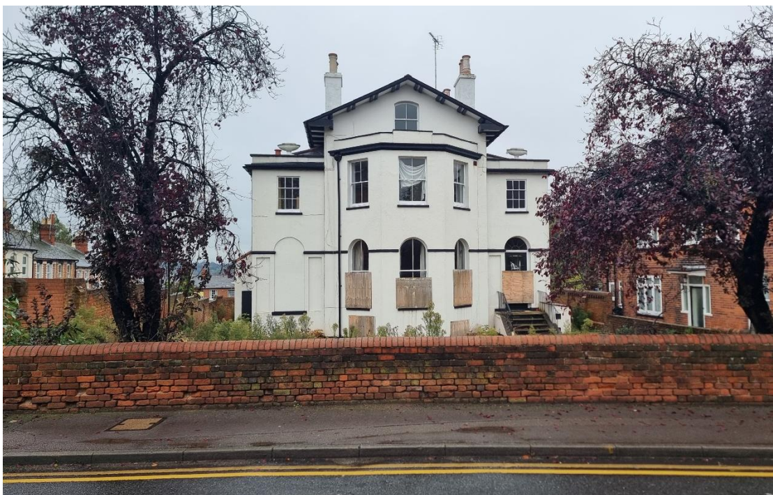
Fig.2: Front (south) elevation of the property, seen from Tilehurst Road.
