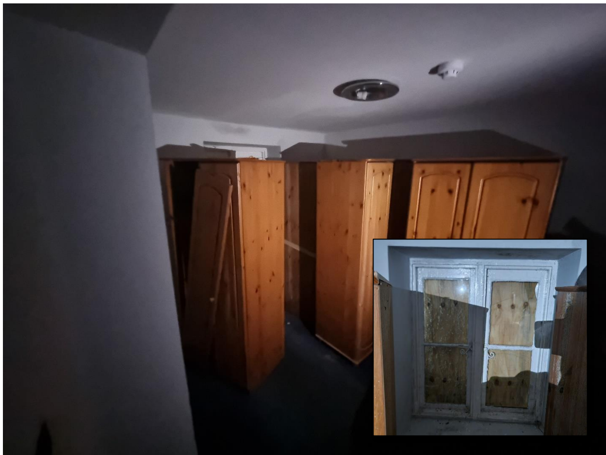
LGF13 - Modern fabric, small casement window of historic context with modern glass
