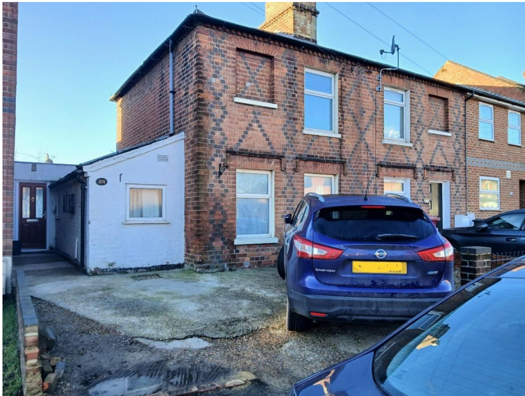
Front Elevation of existing as seen from Gosbrook Road, Reading
