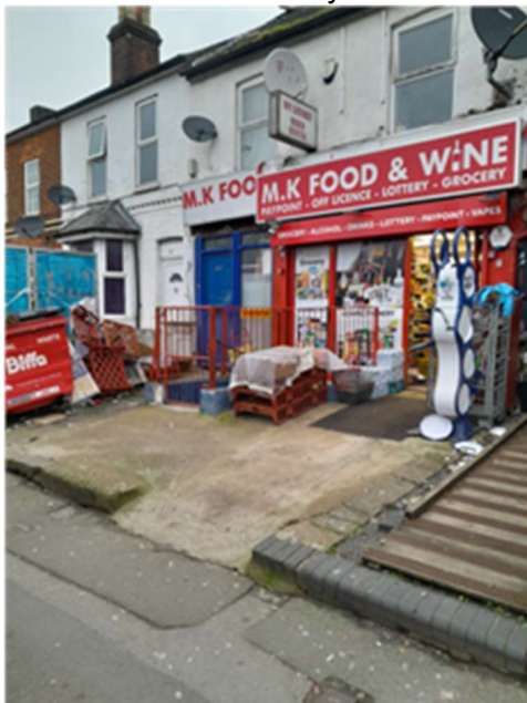
Front elevation, showing proliferation of clutter and existing shop front with new and old illuminated signs and wall mounted projecting sign.
