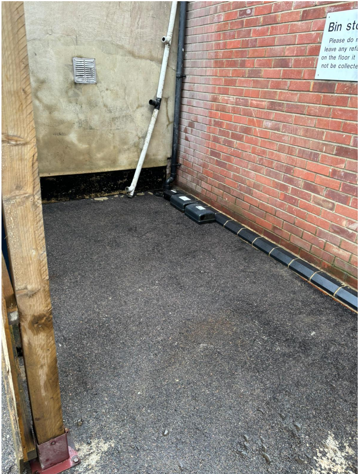
Existing Bin Store Empty
