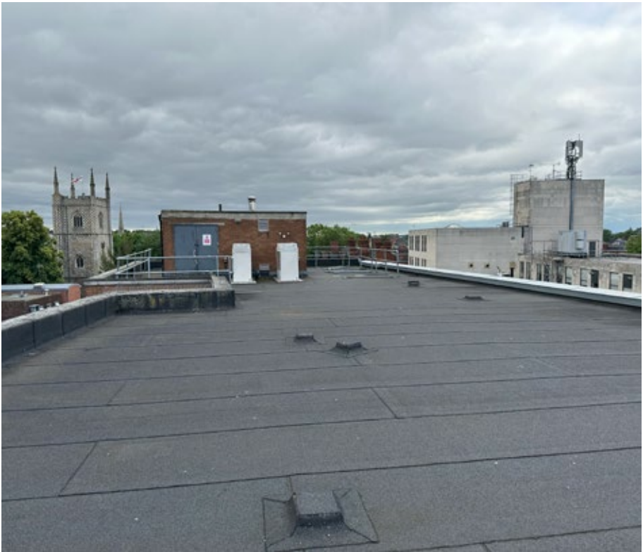
P.16 View from the roof looking south.
