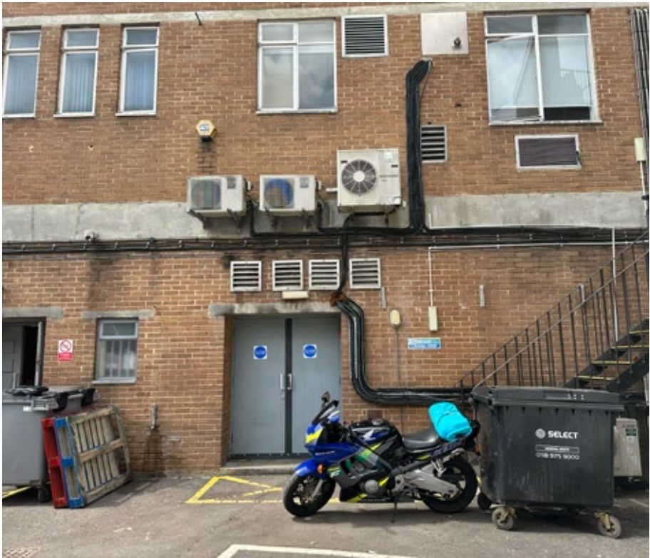
P.12 View towards the rear (East) facade.
