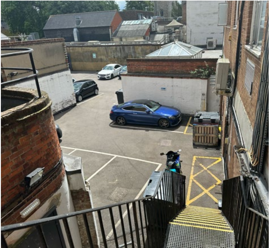
P.11 View from the rear M.O.E. over the carpark.
