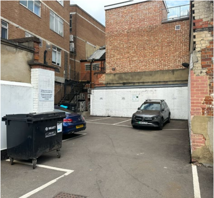
P.15 View towards the rear (East) facade and M.O.E.
