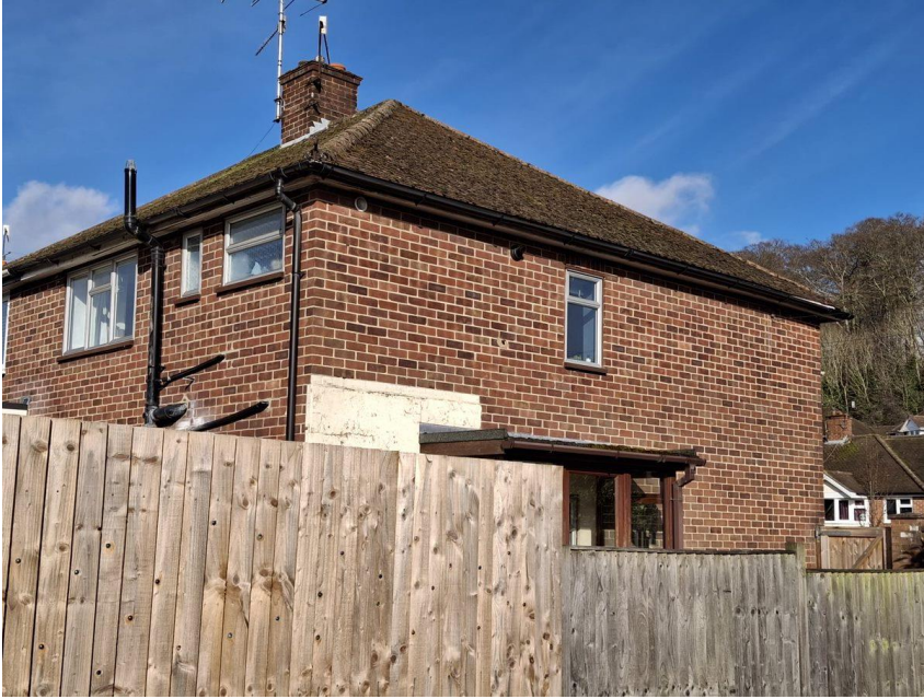
Figure 4: The rear (west) and side (south) of 340 Hemdean Road
