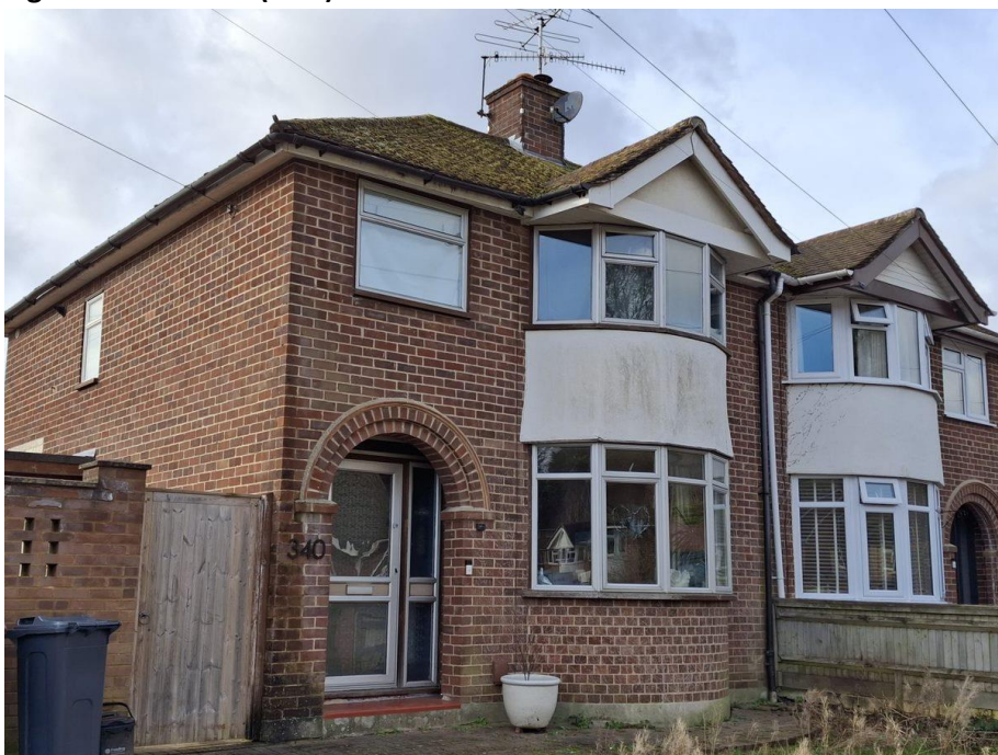
Figure 3: The front (east) of 340 Hemdean Road
