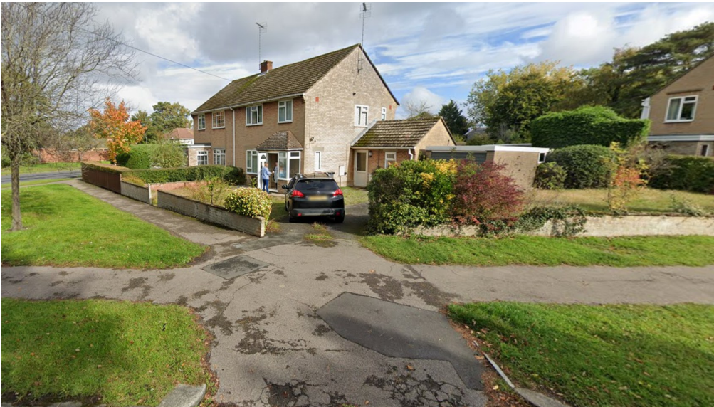
Fig.01 View of the site
