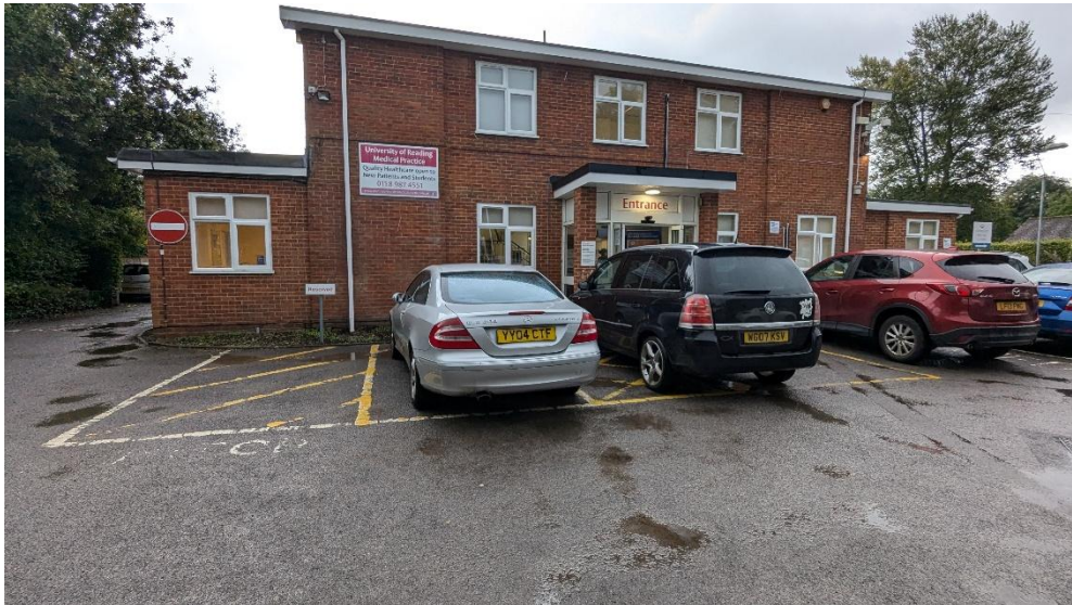
Figure 2.1 View of main entrance and existing disabled parking space
