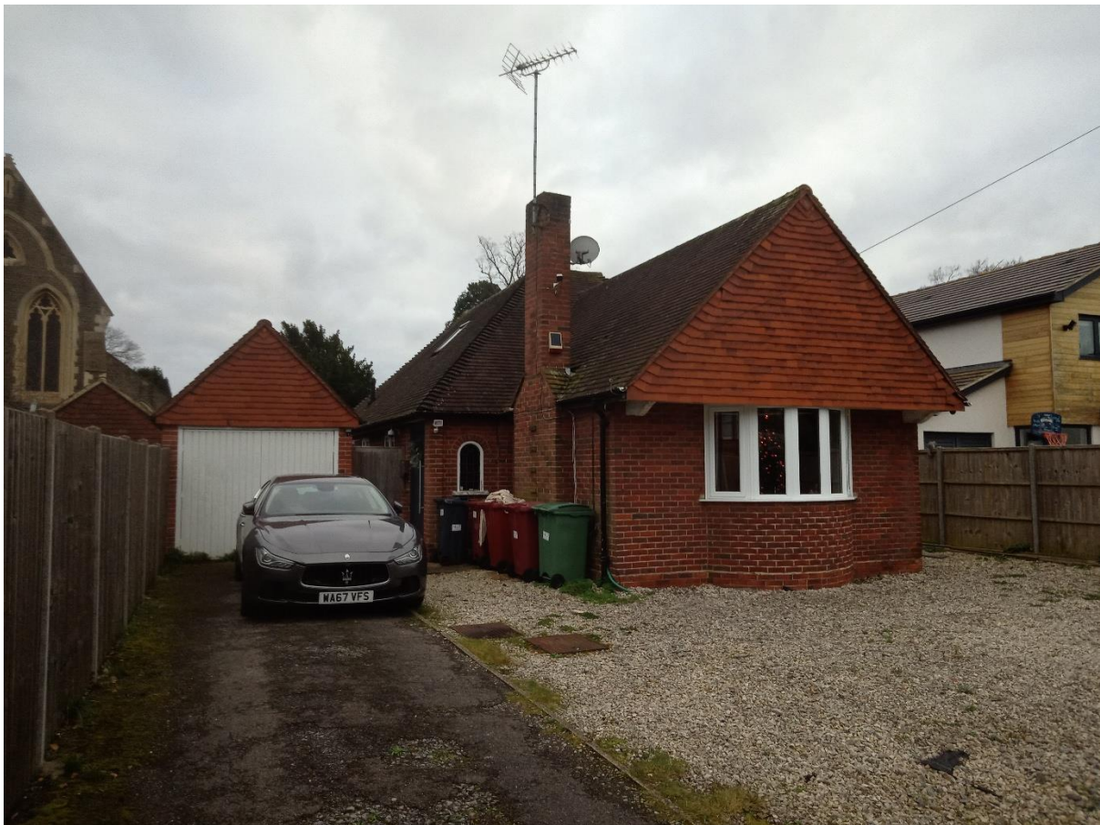
Figure 1 - Picture of Front Elevation
