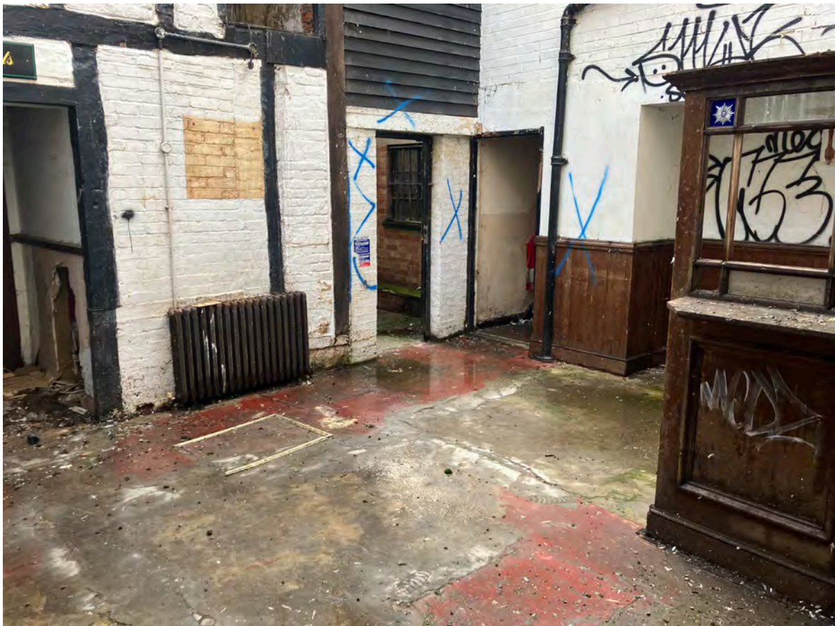
Plate 2: View of Existing Internal Courtyard Area
