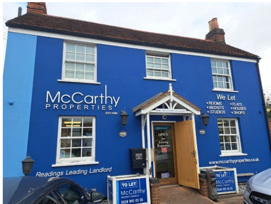
Photo 1 – View of front (south) elevation
