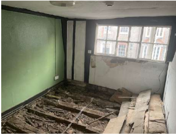
Figure 15: The floor joists can be confirmed to have failed structurally; Figure 16: The timber joists on first floor can be confirmed to have weathered and deflected;
