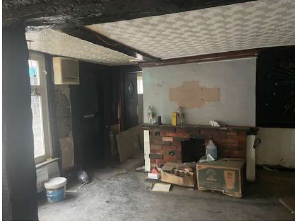
Figure 27: There ceiling can be confirmed to have encountered deflection due to the age of property; Figure 28: The collapse of ceilings area on ground floor due to egress of water;
