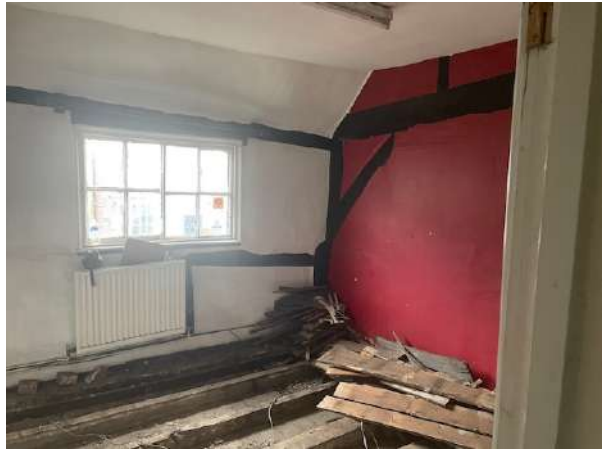
Figure 15: The floor joists can be confirmed to have failed structurally; Figure 16: The timber joists on first floor can be confirmed to have weathered and deflected;
