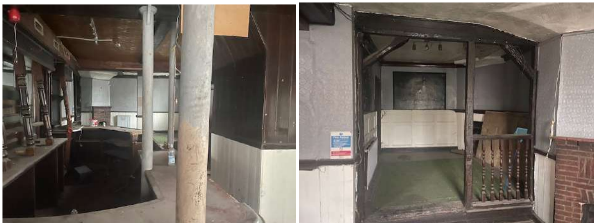
Figure 23: There steel post around the bar counter area can be confirmed to be good condition; Figure 24: The timber post and timber post was found to be adequate;
