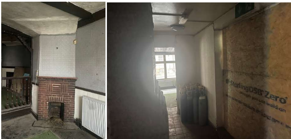
Figure 25: There brick chimney was found to be structurally adequate and timber beam free from any defect; Figure 26: The corridor area on ground floor can be confirmed to be satisfactory;
