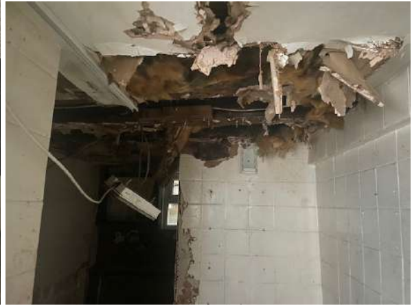
Figure 27: There ceiling can be confirmed to have encountered deflection due to the age of property; Figure 28: The collapse of ceilings area on ground floor due to egress of water;
