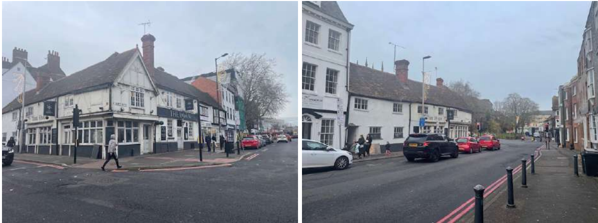
Figure 3: Front and Side Elevation can be confirmed to have signs of ageing and weathering; Figure 4: The Side Elevation rendered developed in early 20 th century was found to be in fair condition.
