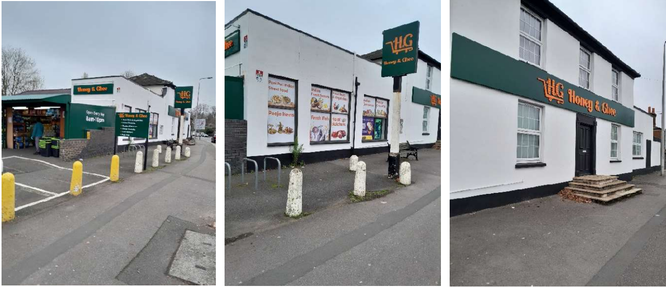
Looking north-westerly towards front elevation
