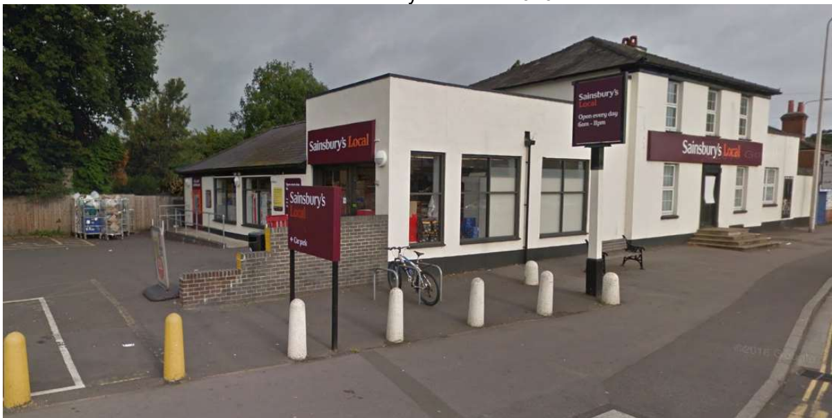
Looking north-westerly towards front elevation
