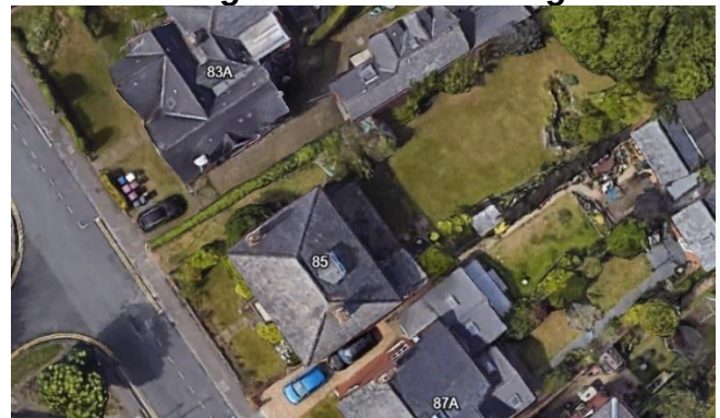
Google Earth Aerial image
