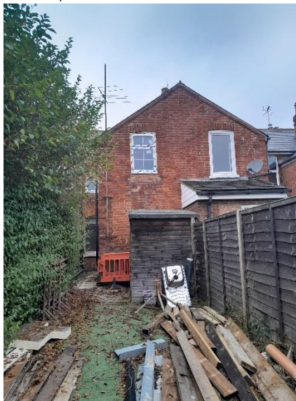
Fig 1: Site photo from the rear of the property, captured by officer on 17/01/2025
