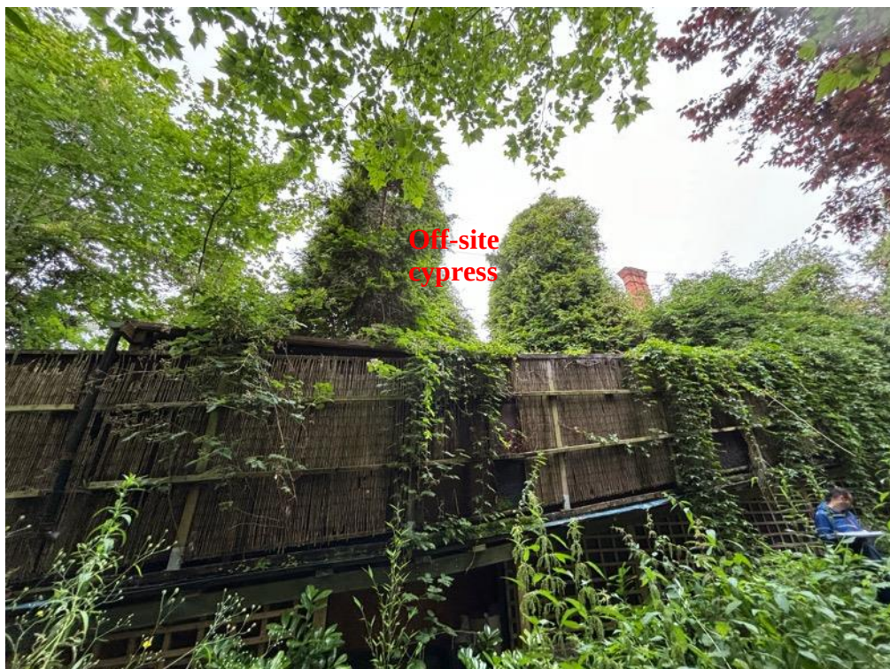
Photoview 6: View west at the raised timber walkway.
