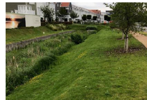
On site storm water attenuation
