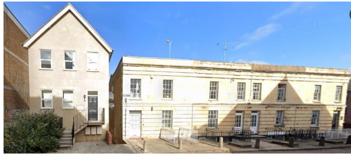
Existing listed terrace
