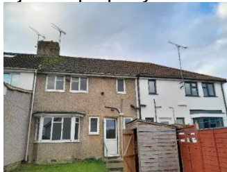
Fig 1: Site photo from the rear of the property, captured by officer on 14/01/2025
