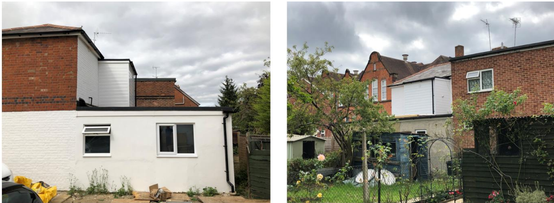
Figure 2 - 2019 photos from rear and side of no.5 Wilson Road
