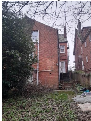
Fig 1: Site photo from the rear of the property, captured by officer on 23/12/2024
