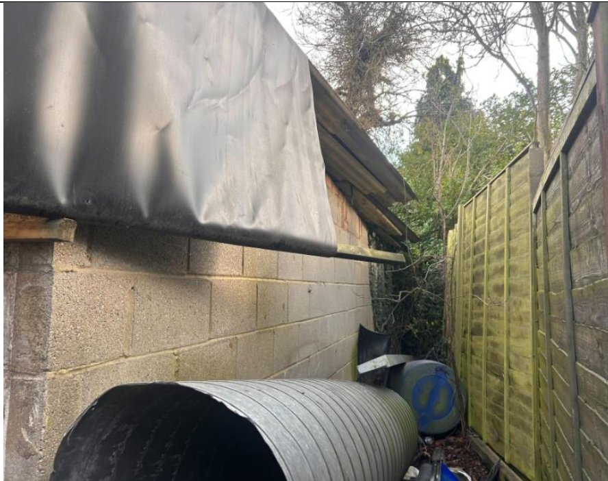
The southern elevation of B2
