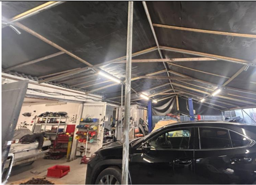
The western elevation of B2
