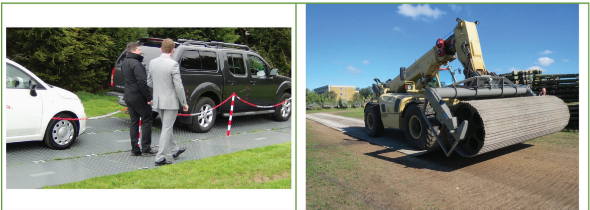
Fig.2: Examples of track board ground protection systems – specification will be dependent on the loading to which it will be subject.
