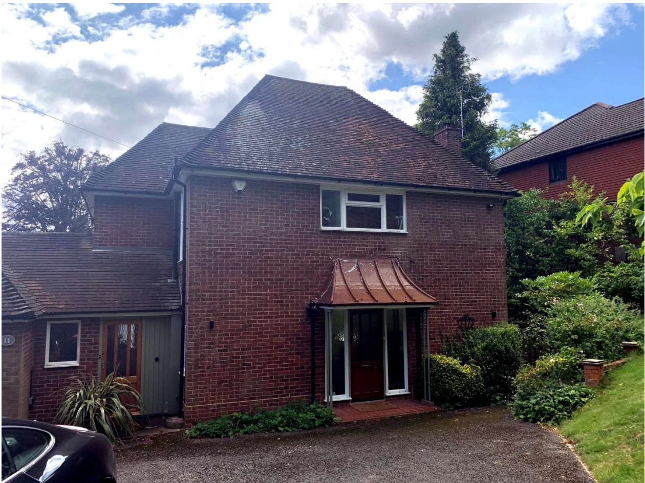
PHOTO 918.1-03 (C IMG_9135): View from NE from driveway.
