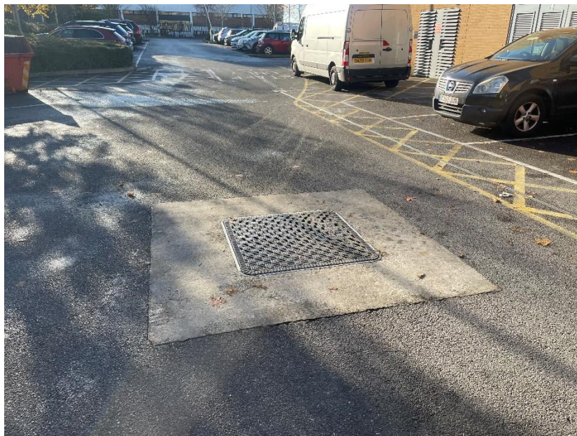
Existing Underground Fuel Tank Location
