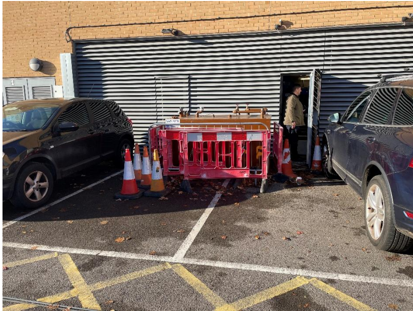
Temporary External Fuel tank
