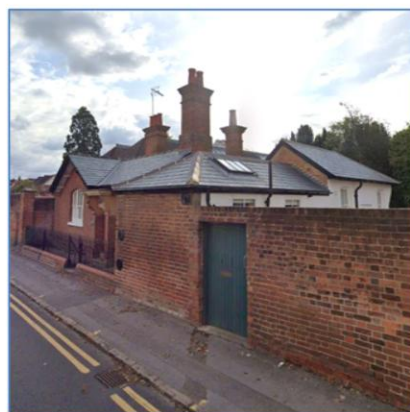
Fig 2. 2 Redlands Road. Image captured in October 2020 following replacement of roof. Image retrieved from Google Maps on 09/09/2022.
