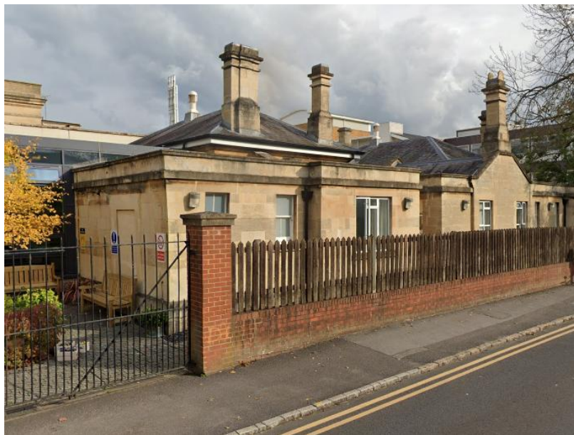
Figure 12 - Screenshot from Google Maps of Royal Berkshire Hospital on opposite side of Redlands Road.
