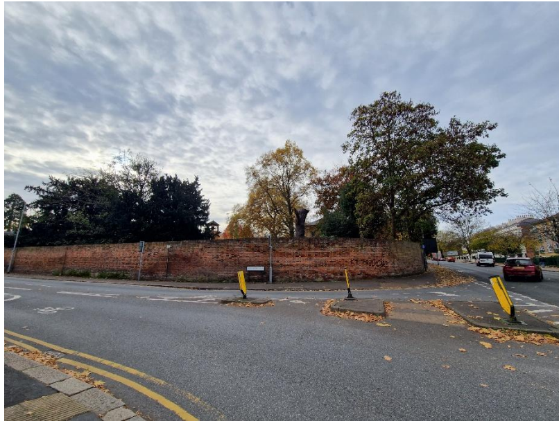
Figure 5 - Listed wall at junction between Redlands Road and London Road
