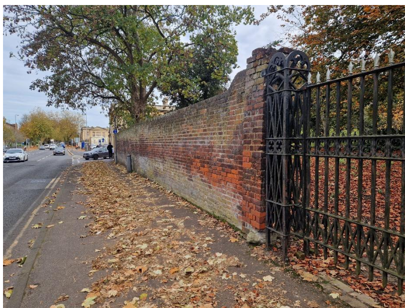
Figure 4 - View along London Road of the listed wall to The Acacias.
