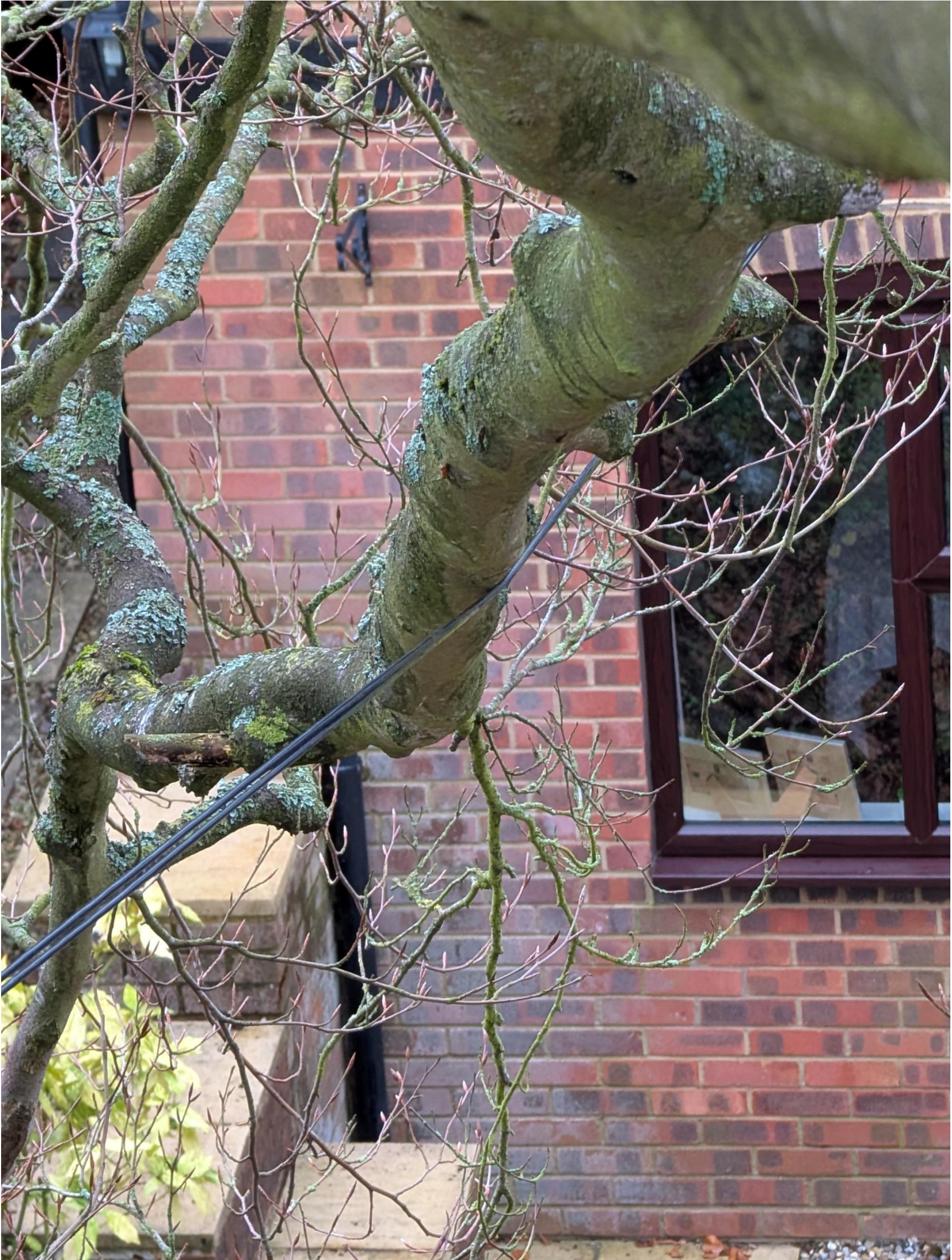
B.7 – Limb rubbing on phone cables over front garden side (South) approximately 7m.
