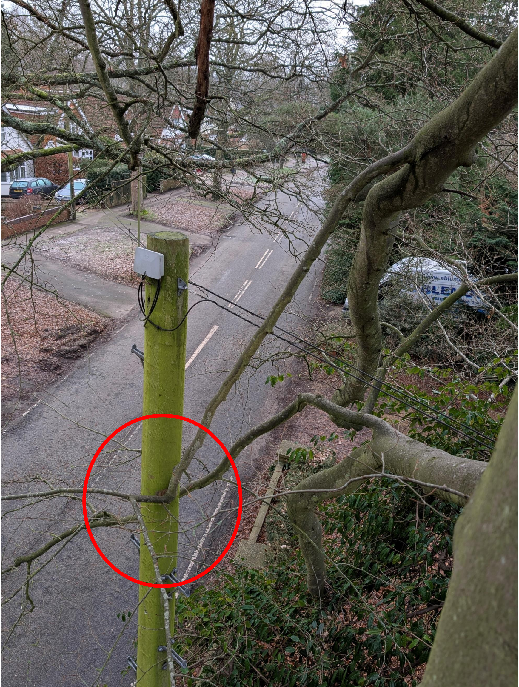
B.6 – Multiple limbs in close proximity to the telephone cable pole. Highlighted limb rubbing on pole.
