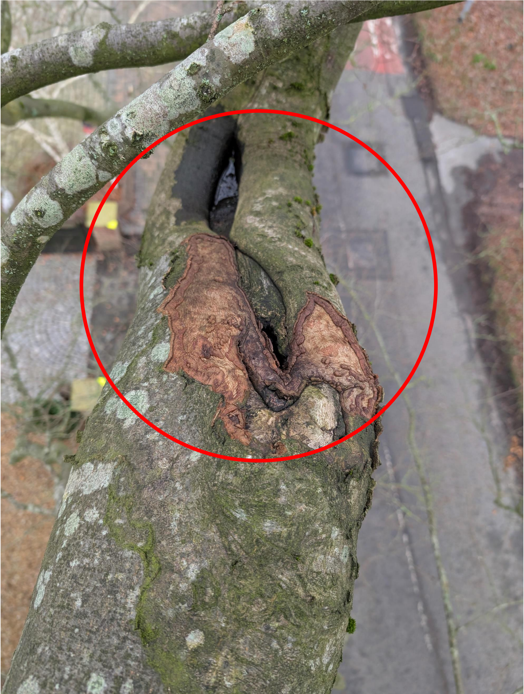
B.5 – Image of decay and squirrel damage at 11m on north stem lateral limb.
