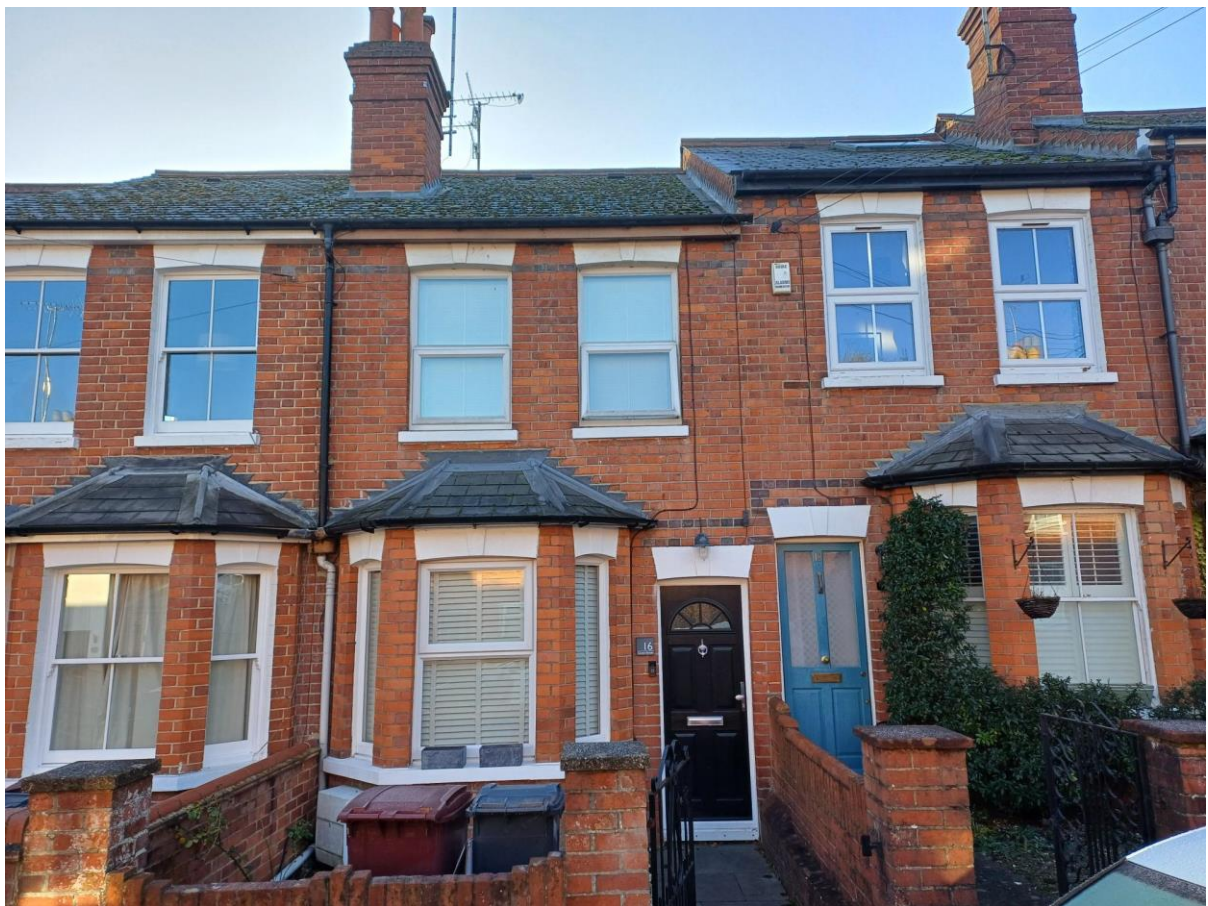
Site Visit Photos taken on 9 th of January 2025
