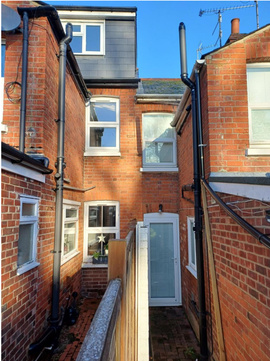
Site Visit Photos taken on 9 th of January 2025
