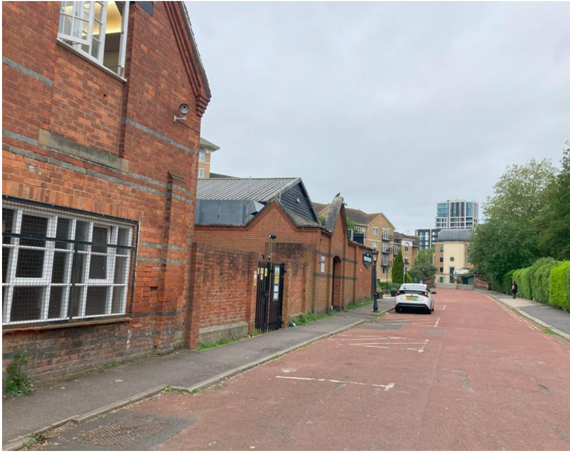
Above – View looking southwest along Gas Works Road with location of louvres hidden within recessed façade elevation of the former pumphouse
