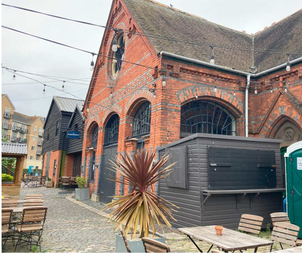
Above – View of southeast and northeast existing windows
