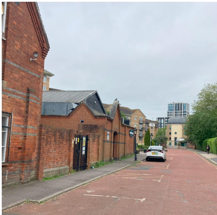
Above – View looking southwest along Gas Works Road
