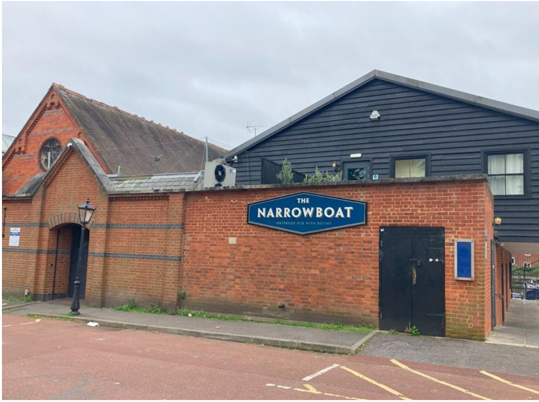
Above – View of existing Gas Works Road elevation
