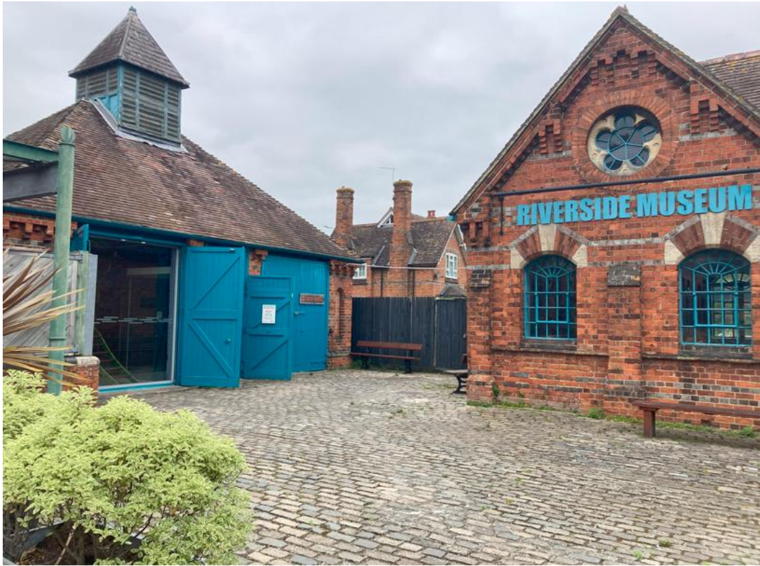
Above – View of river front access to adjacent museum
