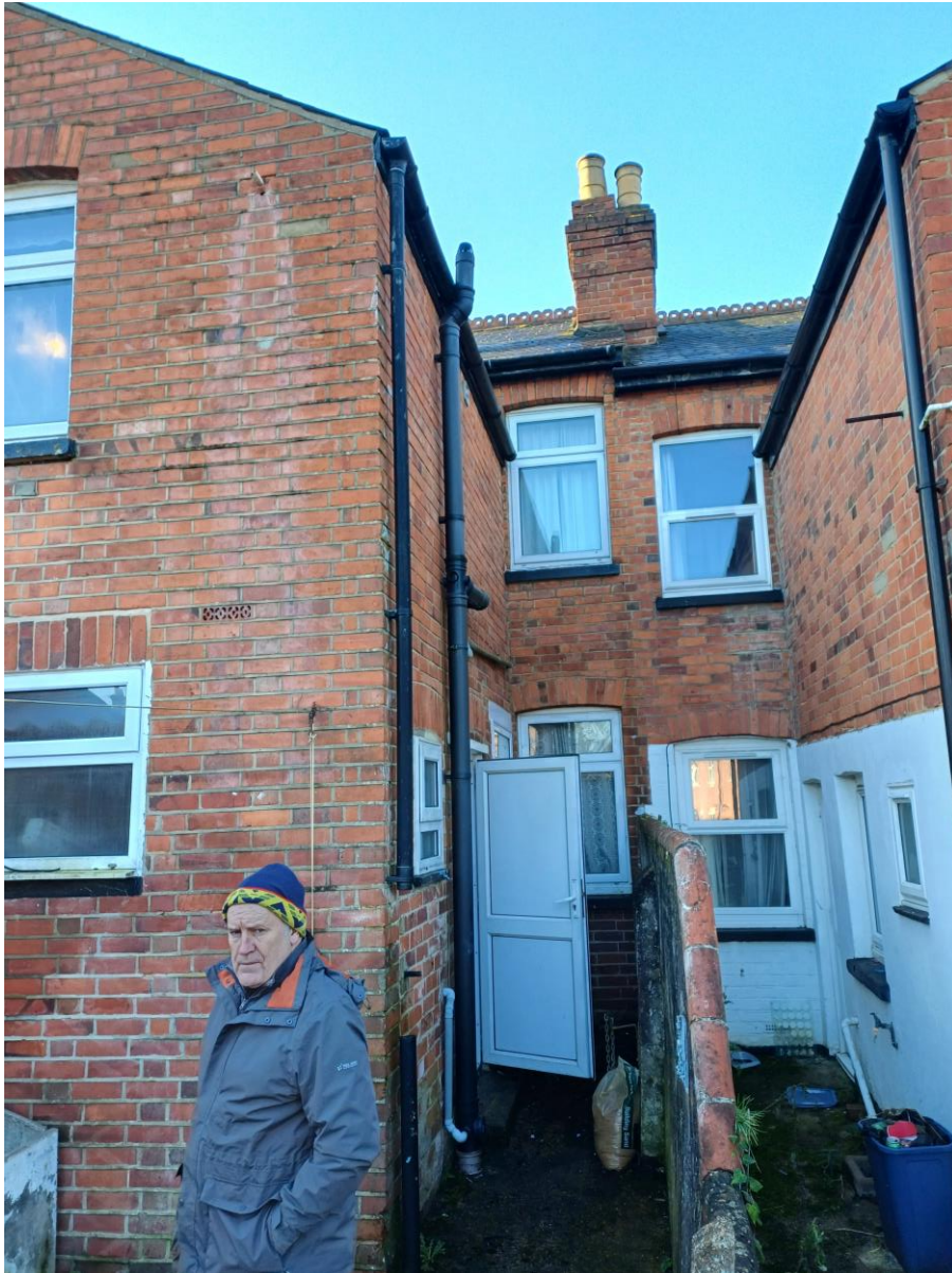
Site Visit Photos taken on 9 th of January 2024
