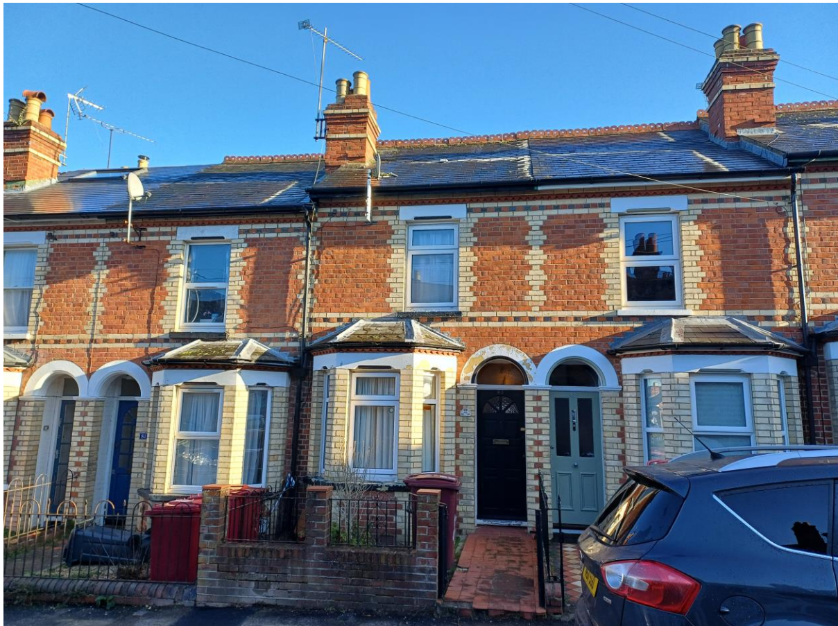
Site Visit Photos taken on 9 th of January 2024
