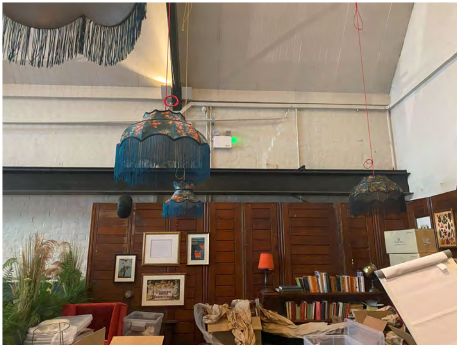
Plate 16 – Southwest elevation looking towards area where new opening is to be formed at high level with existing metal beams and pipework present.
