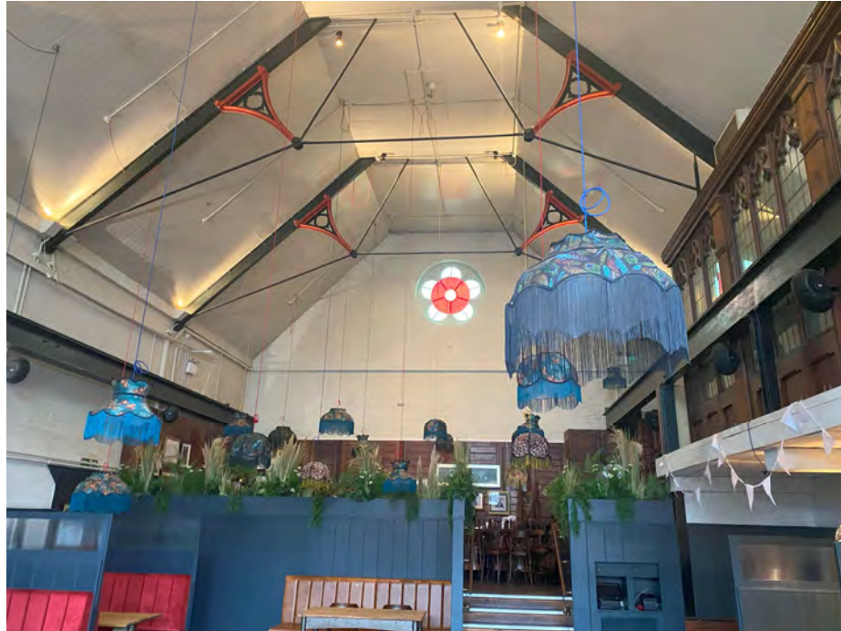
Plate 14 – View through the interior space with existing metal columns and beams and roof trusses.
