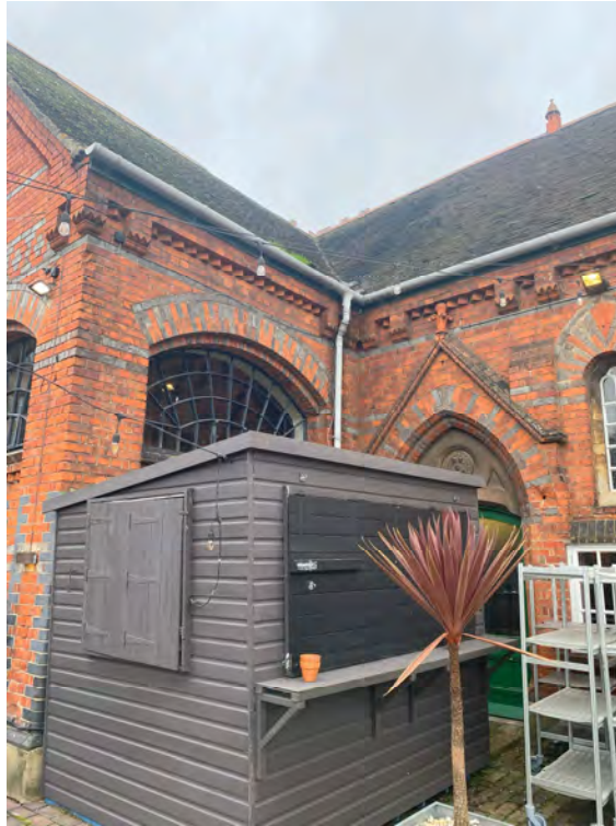
Plate 13 – Overlight to be temporarily altered on the southeast frontage.
