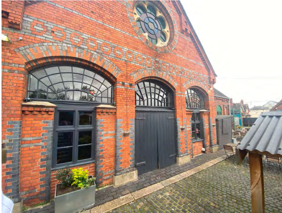
Plate 11 – Southeast frontage onto Canal.
