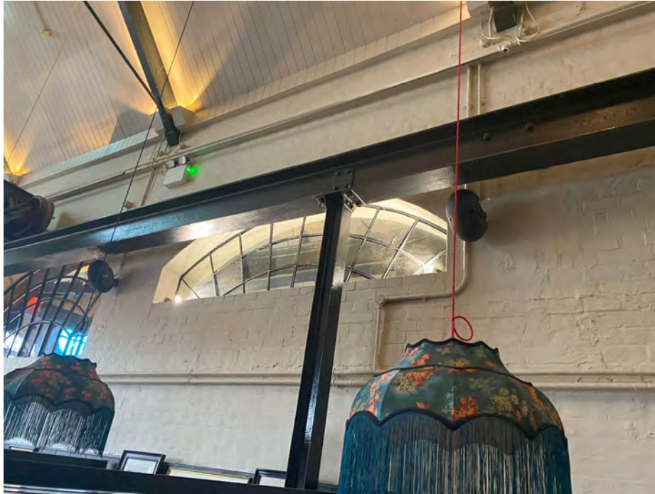
Plate 15 – Existing metal work to interior of the space with painted, exposed brickwork wall and surface mounted pipework and cabling to the southwest elevation.
