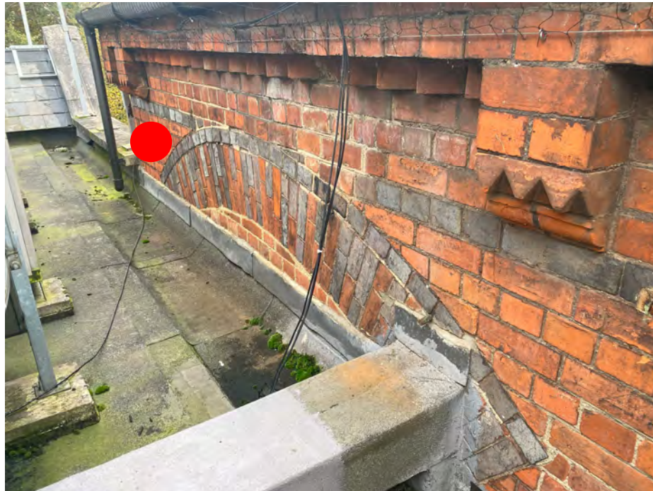
Plate 10 – Southwest elevation of original building and junction with extension; area of proposed opening identified by red circle.
