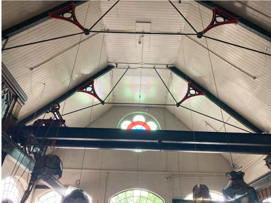
Plate 5 – Metal roof trusses and mechanism retained to the interior.
