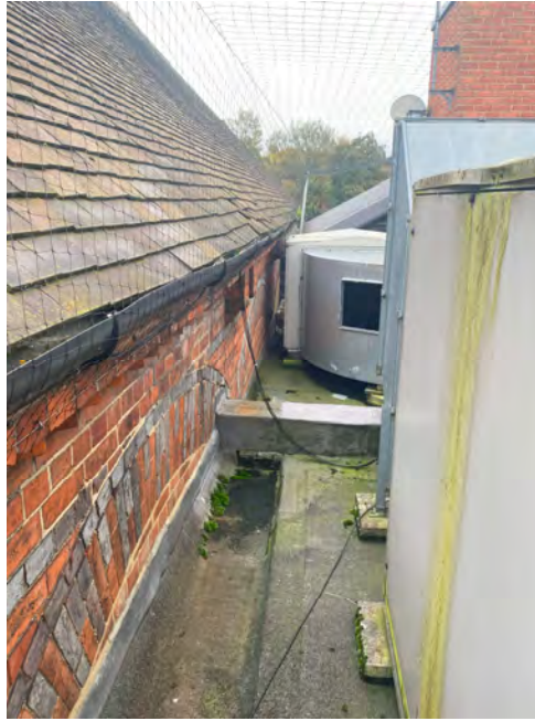
Plate 9 – Southwest elevation of former engine house viewed from modern flat roof with corbel table and decorative brickwork to high level
