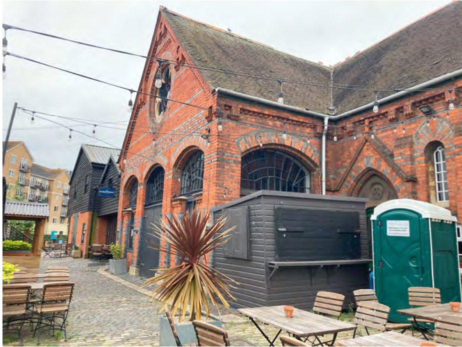
Plate 1 – Left (southwest) block of the Grade II listed former engine house.
