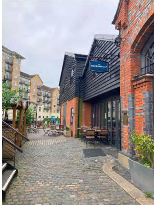
Plate 3 – Later, additions to the southwest which accommodate the majority of the pub and restaurant.
