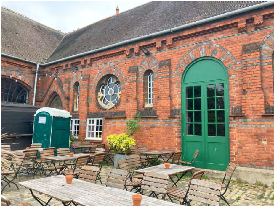
Plate 2 – Right (northeast) block of the Grade II listed former engine house.
