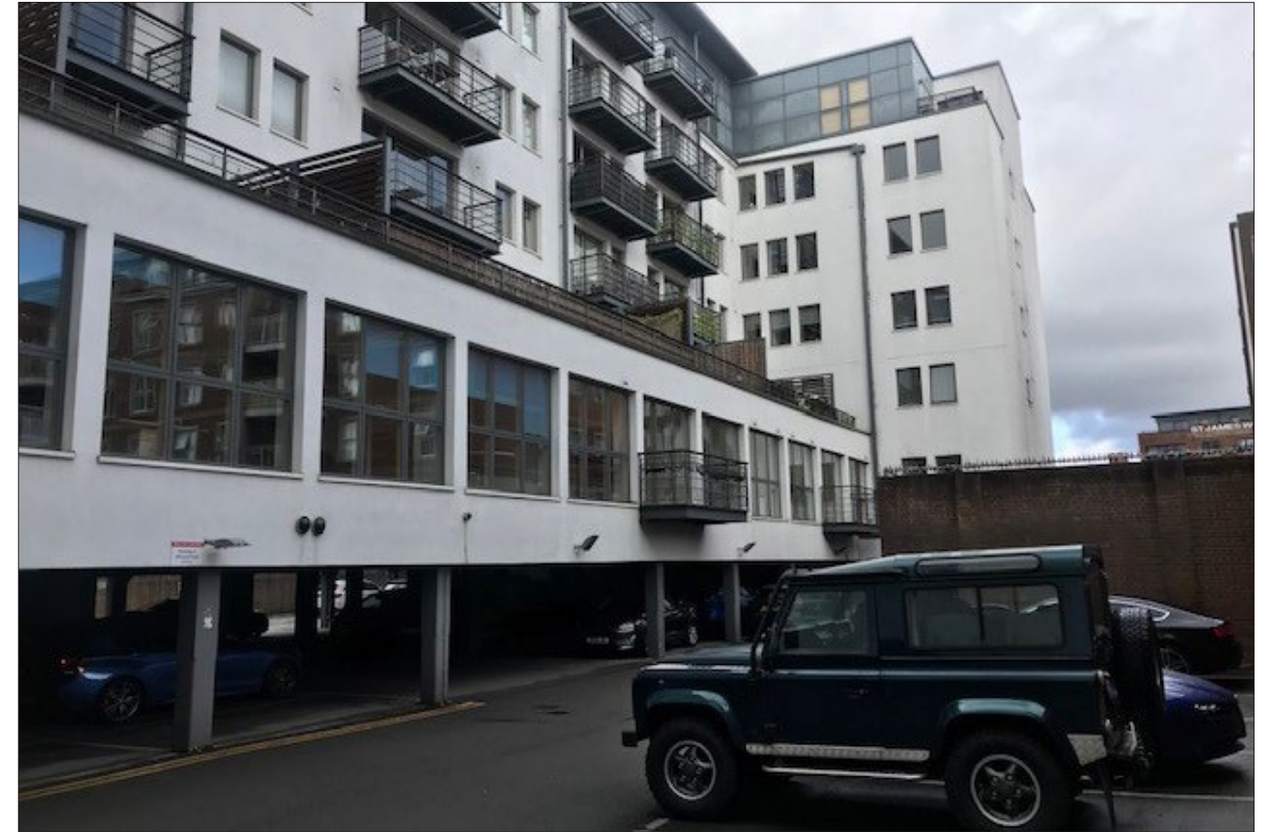
Fig. 9 First Floor units facing the car park. Private residential balconies and terraces can be seen at upper floors
