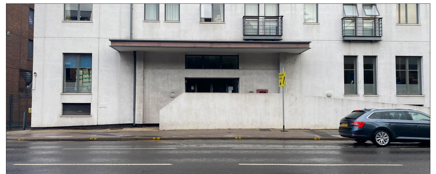
Fig. 11 Principal entrance to the existing ground floor offices off Queen's Road
