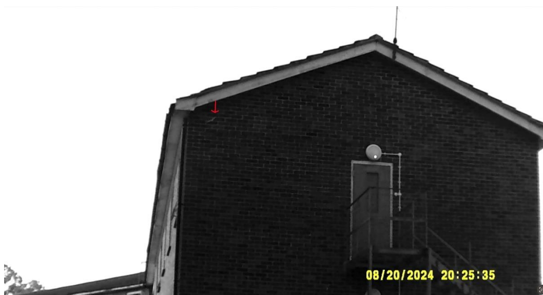
Figure 2 – common pipistrelle emergence on 20 th August from under soffit on south-western elevation.
