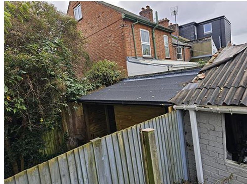
Existing rear extensions – view from site
