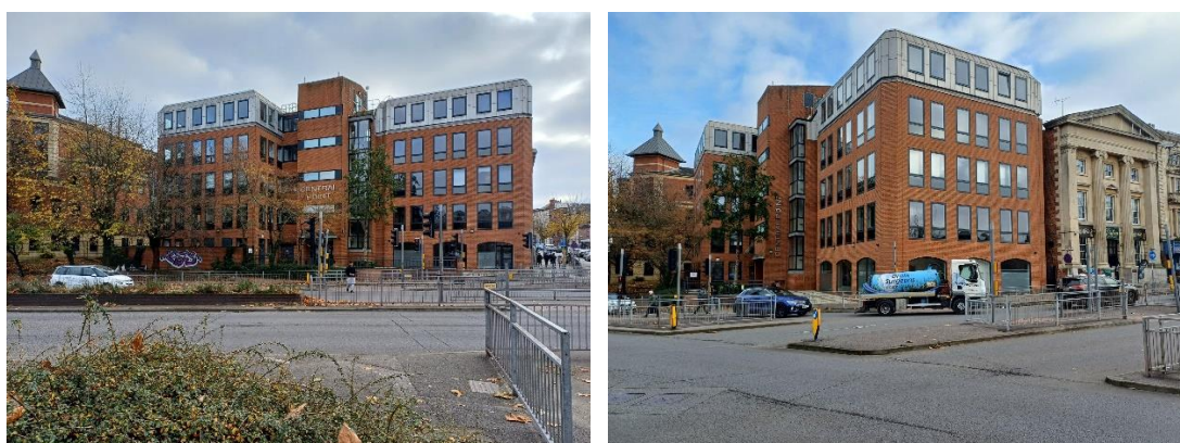
Site photographs 15/11/2024) showing the Queens Road (left) and London Street (right) elevations.
