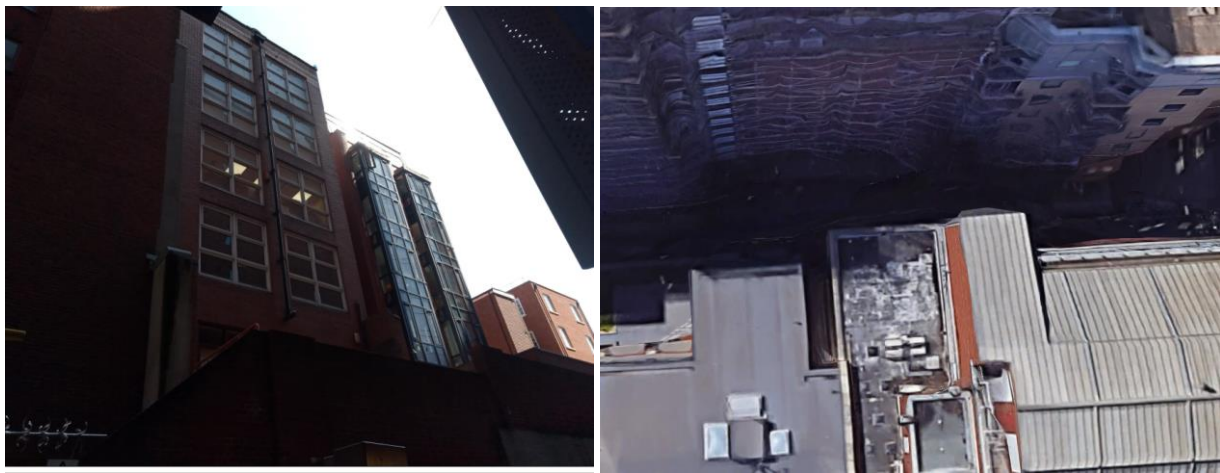
Above: View of the rear of the application site building from ground level & aerial view
