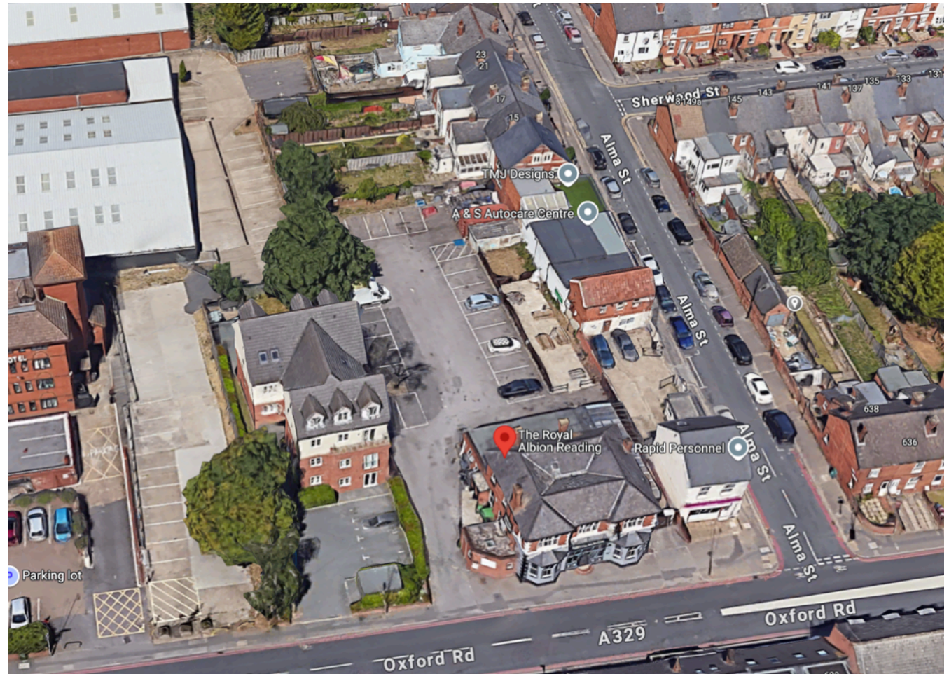
Fig 1: Aerial view of site
