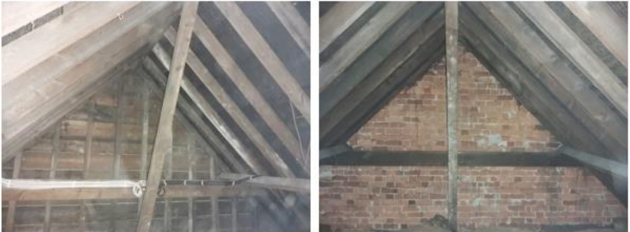
Figure 4: Open loft space showing timber cladding to the south and brick to the north
