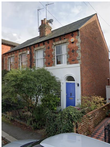
Fig. 1: 36 New Road, captured from Google Street View on 29/11/2024
