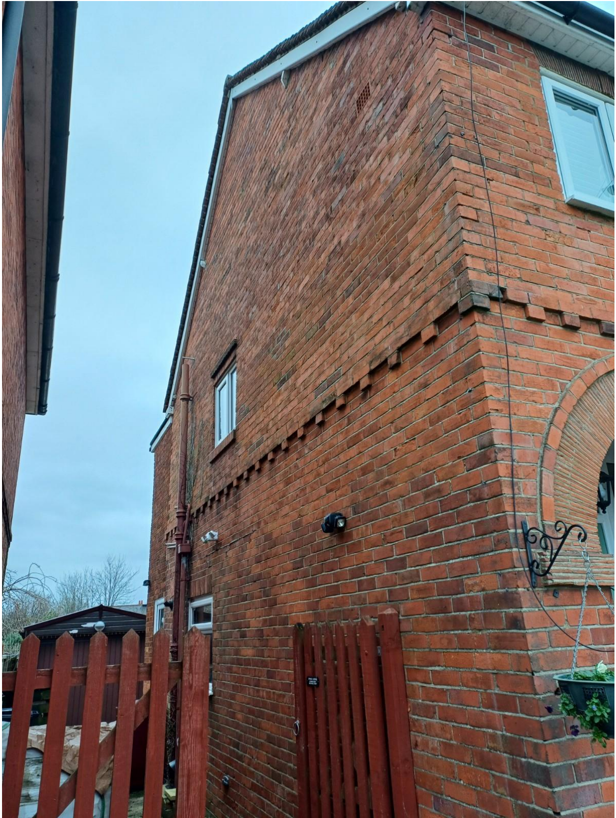
Site Visit Photos taken on 11 December 2024
