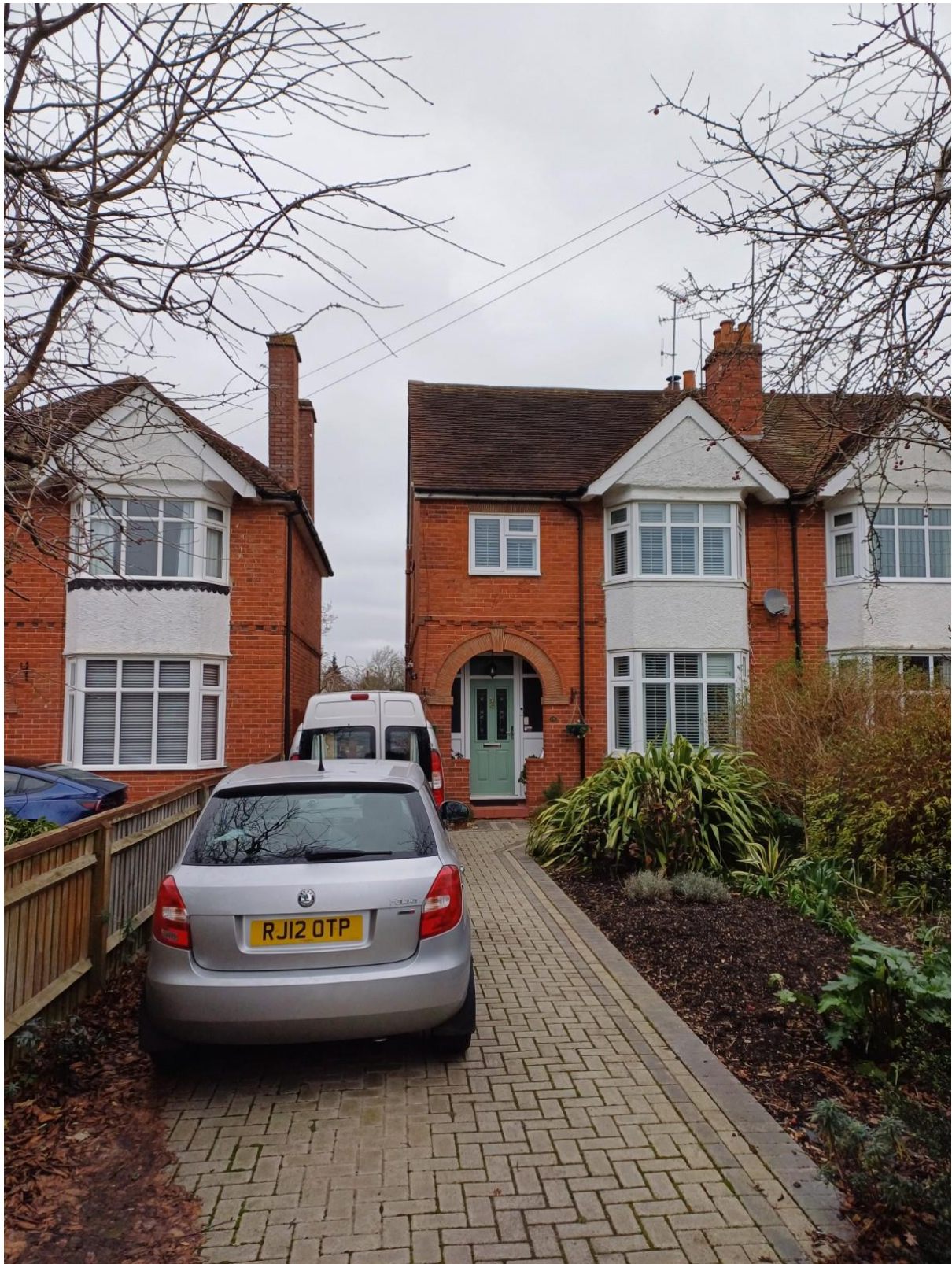
Site Visit Photos taken on 11 December 2024
