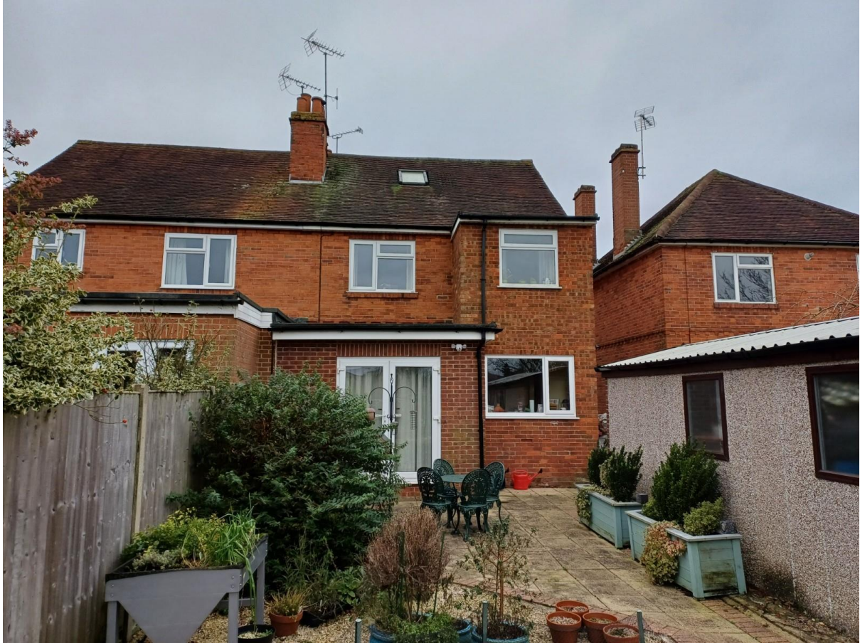
Site Visit Photos taken on 11 December 2024
