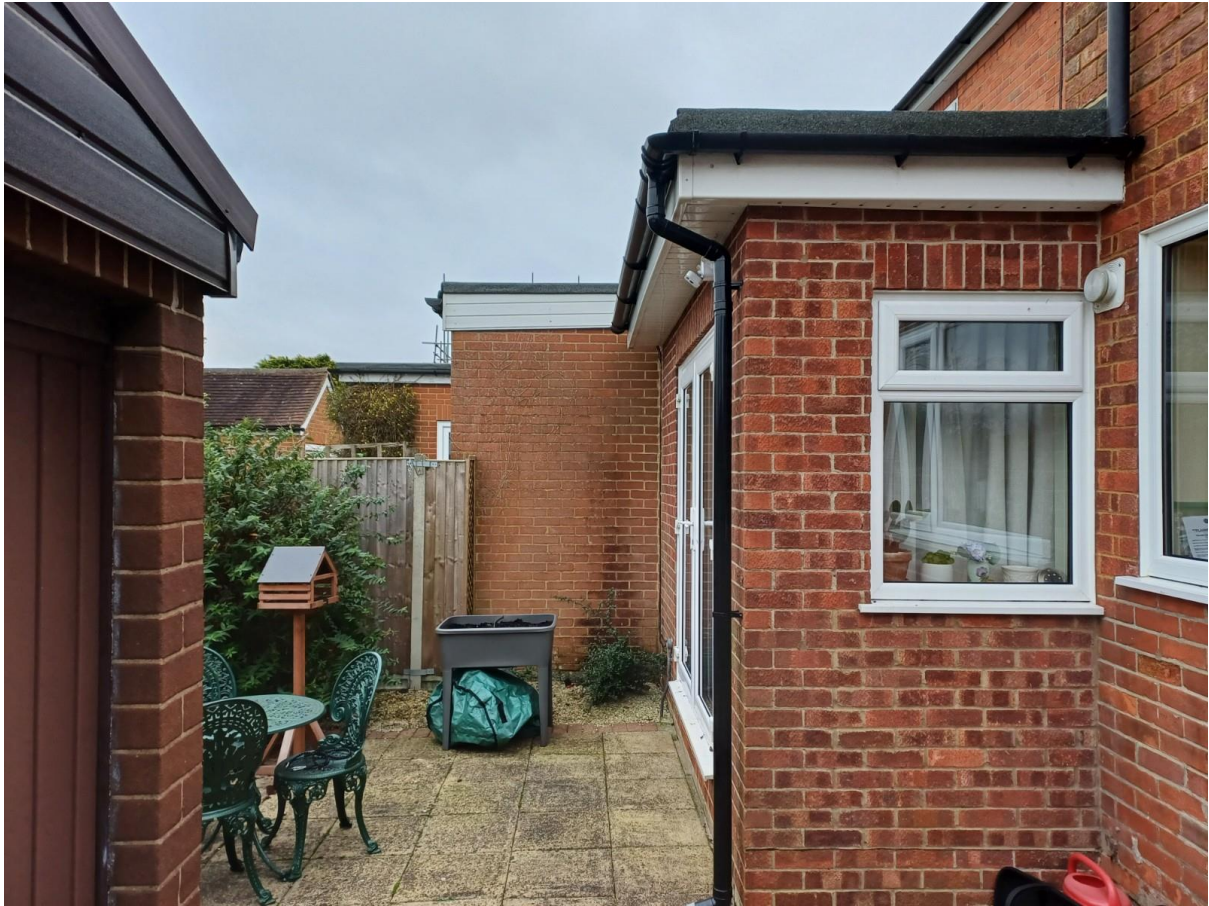
Site Visit Photos taken on 11 December 2024
