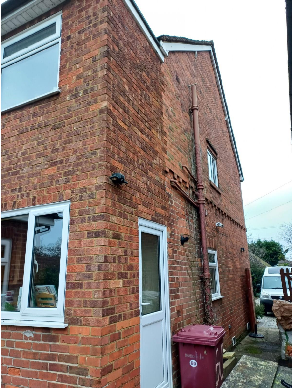
Site Visit Photos taken on 11 December 2024
