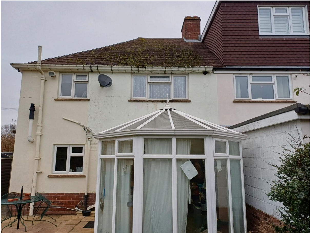
Site Visit Photos taken on 11 December 2024
