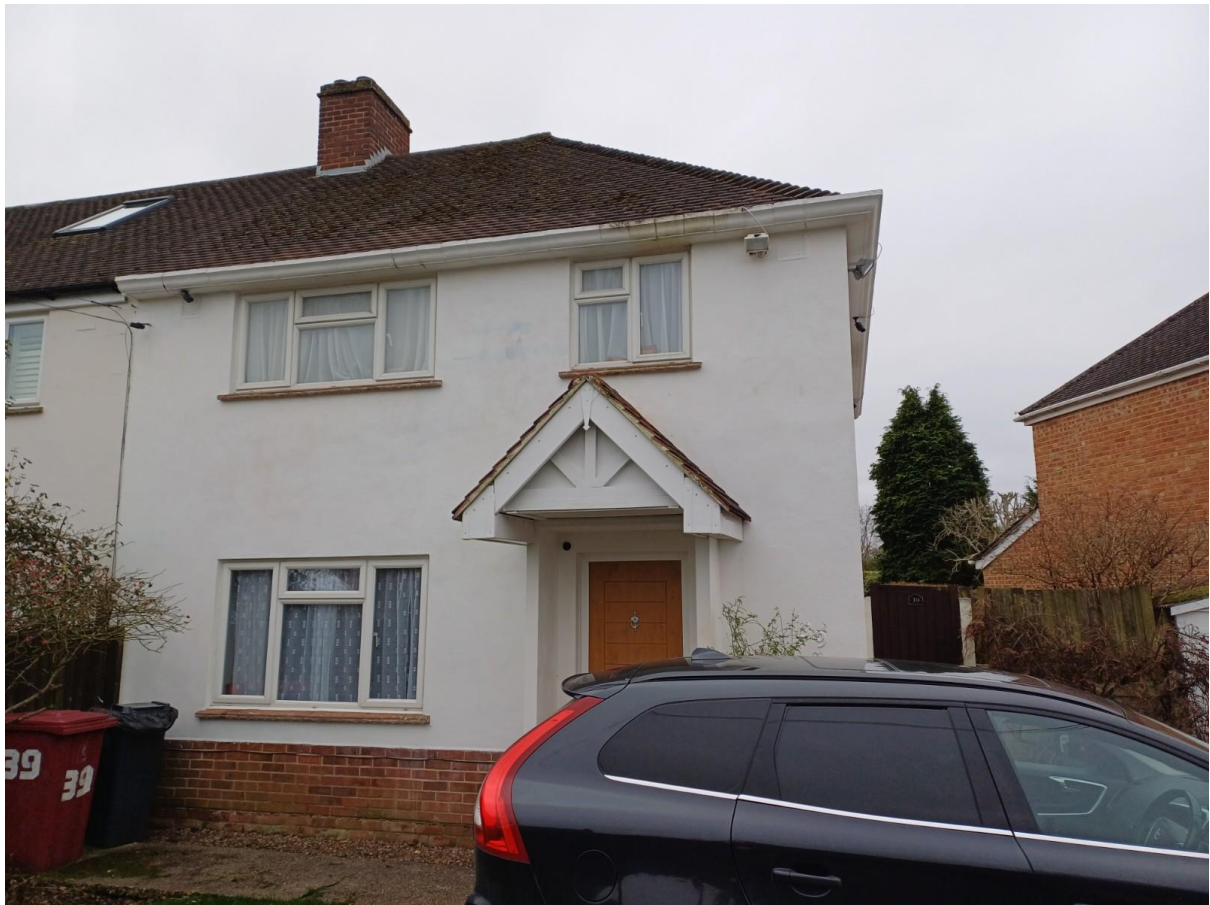
Site Visit Photos taken on 11 December 2024
