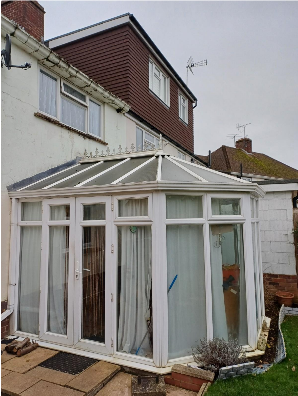
Site Visit Photos taken on 11 December 2024
