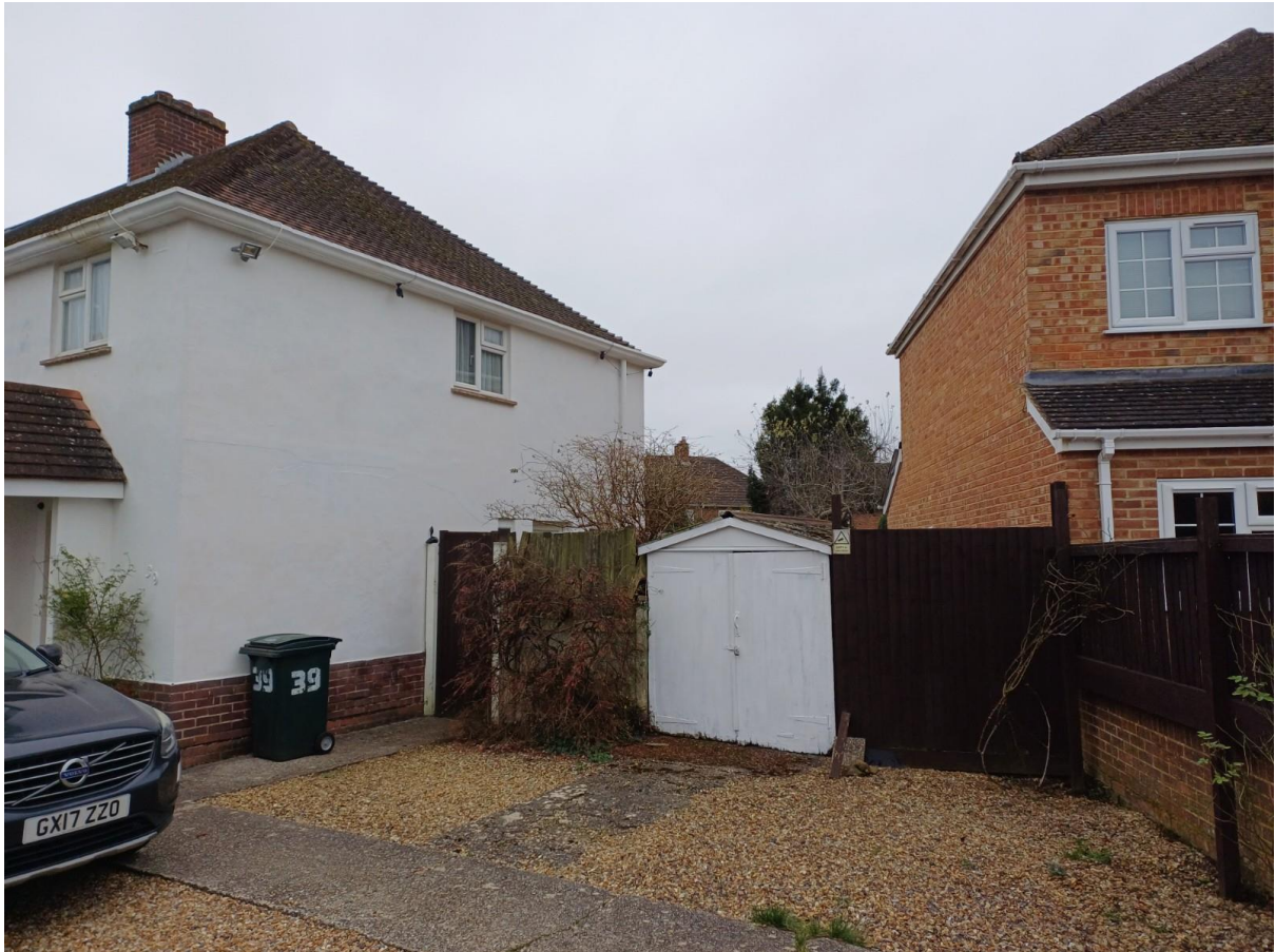
Site Visit Photos taken on 11 December 2024
