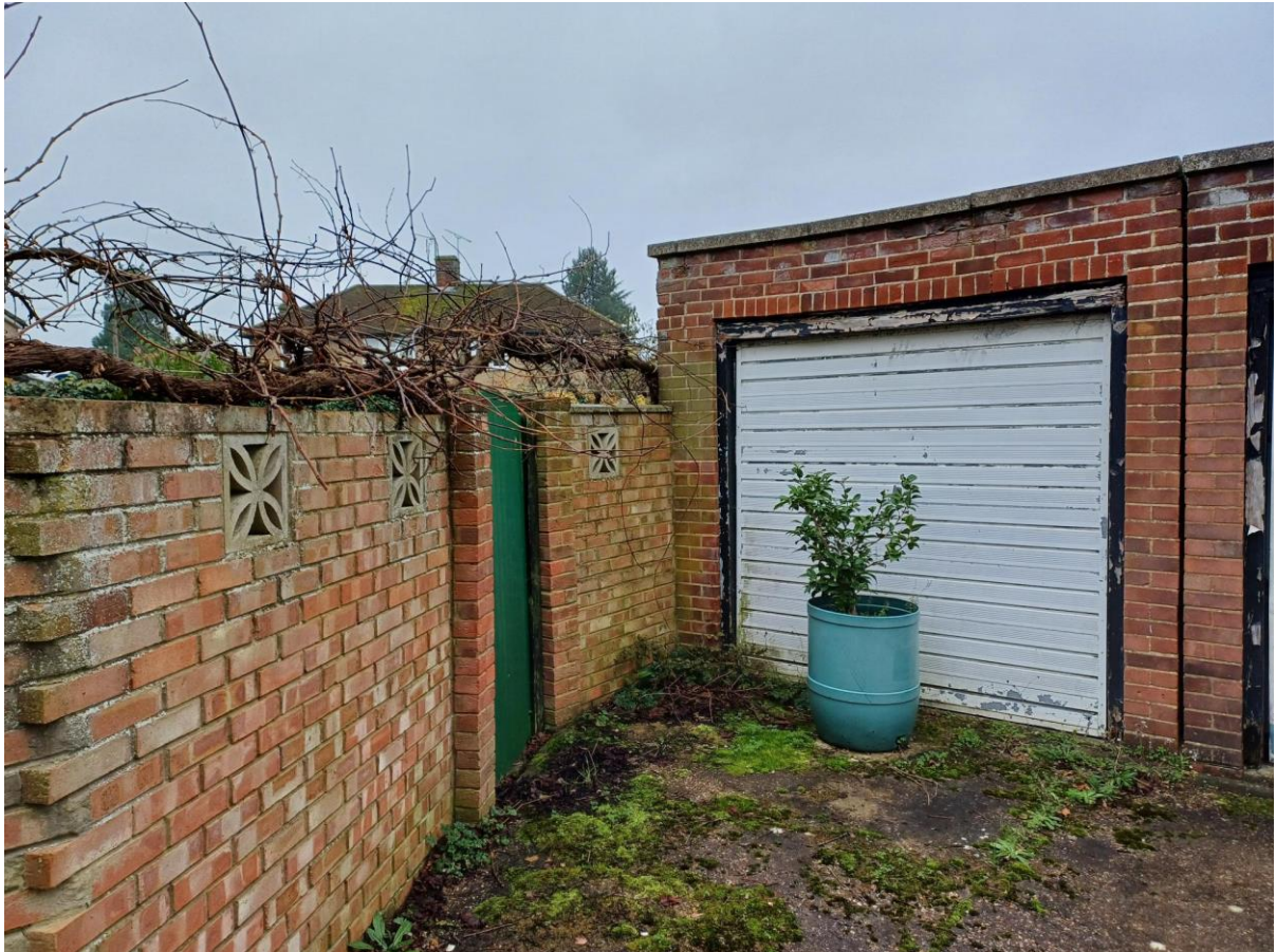
Site Visit Photos on 7 th of November 2024
