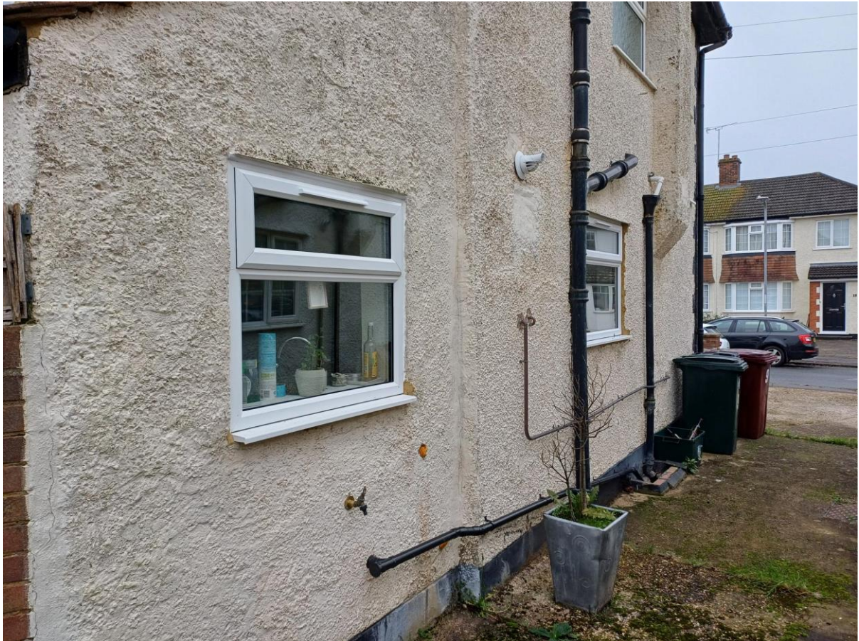
Site Visit Photos on 7 th of November 2024
