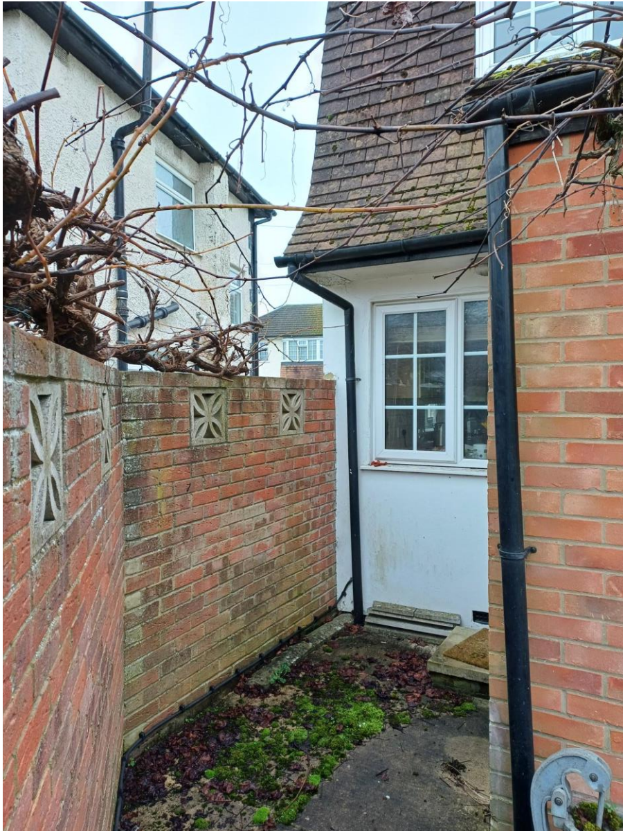
Site Visit Photos on 7 th of November 2024
