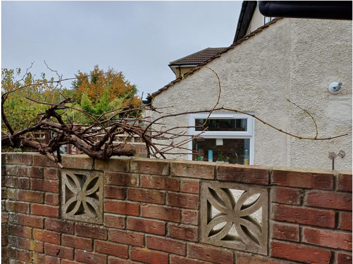
Site Visit Photos on 7 th of November 2024
