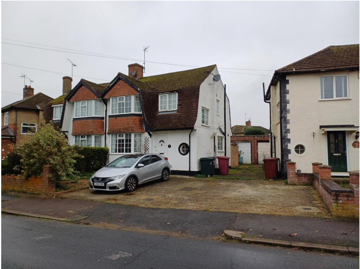
Site Visit Photos on 7 th of November 2024
