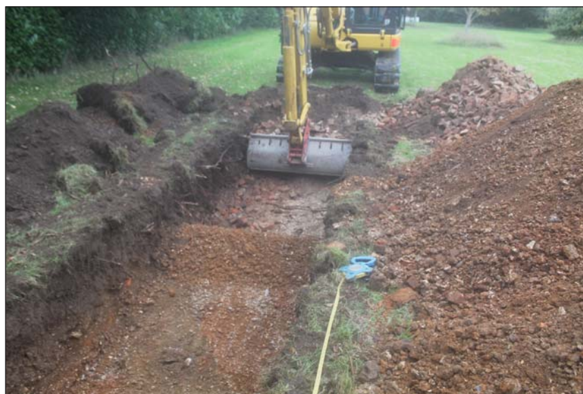
Plate 6. Brick rubble in trench 3, looking West
