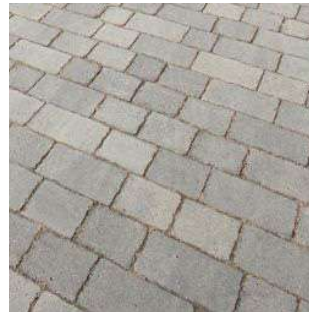
Permeable paving to reduce stormwater runoff volume
