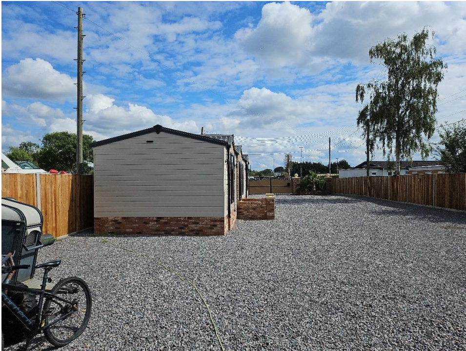
Fig 7. Eastern view across the site. Note the new, prefabricated building on the left. This will be unaffected by the proposed demolition works.
