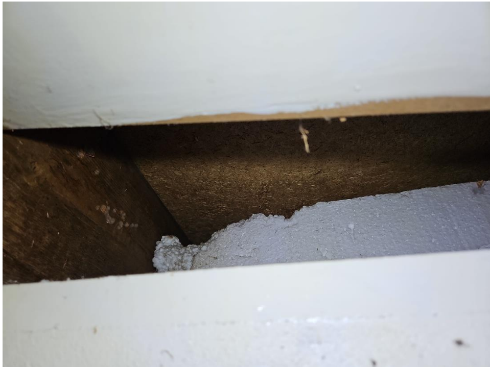
Fig 6. Detail showcasing the limited void space between the bungalow's ceilings and its roof.
