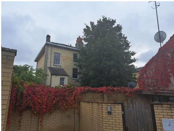
Photo 39 – View of the rear elevation (west elevation) from 43 St Johns Rd.
