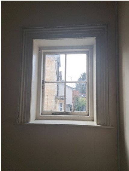
Photo 17-20 – View of the first floor interior (including staircase to second floor)
